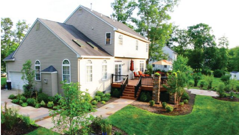
On the completed project, two sets of stairs from the deck to ground level created both visual interest and a more efficient traffic pattern.
