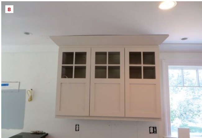
The difference in crown angle can be seen between the wall cabinet in the foreground and the one in the background (6). But when viewed from across the room, the difference is hardly noticeable (7). Slight variations in the ceiling can often be remedied by floating drywall compound down to the level of the crown molding (8).
