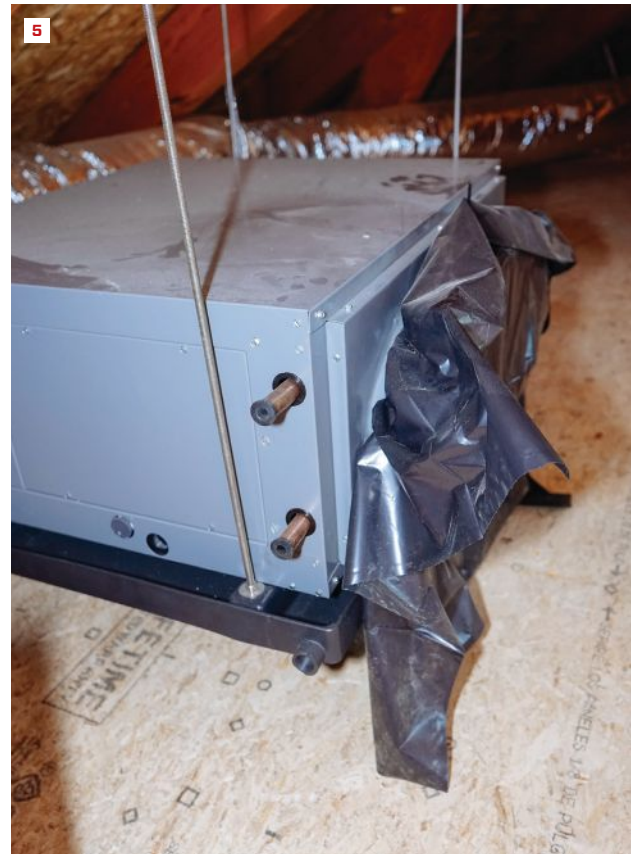
Radiant floors team with hydro-air. ReVision Energy's Chris Blaisdell works on the hydronic tubing for a radiant slab in a custom house (4). Behind Blaisdell is the hydronic buffer tank for the system. On the second floor of this home, a SpacePak high-velocity hydro-air unit (5) will supply heated or cooled air using fluid supplied by the same outdoor-mounted heat pump.
