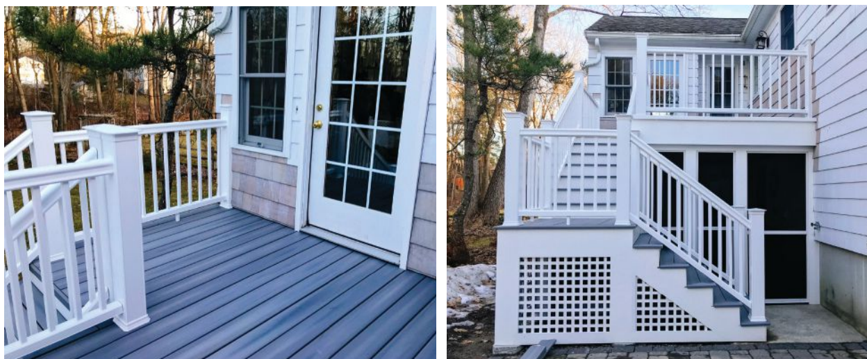
Figure 7. To fit the multiple flashing layers that were used to waterproof the 4x4 guard posts, the author installed composite post sleeves sized to fit 5x5 posts (left). The new deck looks similar to the old one, but has more useful dry space thanks to the new flashing details and new screening that encloses the area underneath the deck (right).
