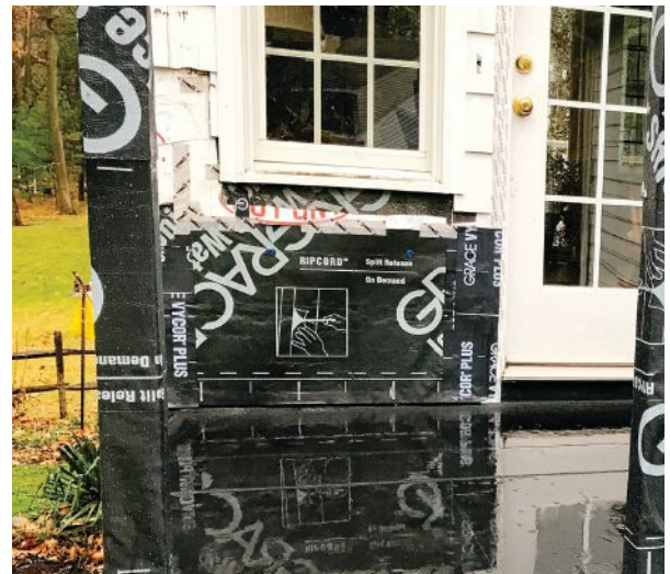
Figure 5. The roof flashing boots were sealed to the posts with Siga Wigluv, a high-performance tape (top right), then the posts were wrapped with SAF flashing membrane (bottom right).
