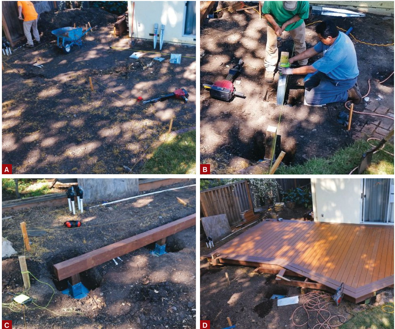
Figure 4. Oz-Post bases are typically installed on-grade using a jackhammer and a special bit that fits inside an insert placed in the base (A). On this project, the post bases were placed in shallow excavations (B) to keep the carrying beams close to ground level (C). The author typically limits his use of Oz-Posts to low freestanding decks on level ground, like this one (D).
