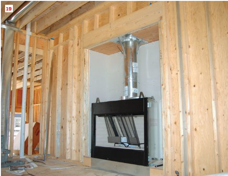
Fireplace inserts are typically boxed into framed recesses that leave open framing areas connecting the conditioned space with the exterior (18). A good solution is to build a sealed chamber for the insert (19). The chamber will be hidden once drywall is hung on the walls.
