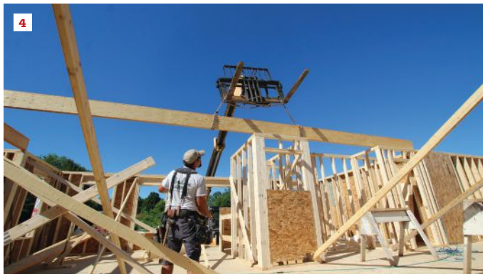
The 32-foot-long beam is built safely on the ground (1). The longer LVLs are chained to the telehandler's forks, ready to be moved (2). The telehandler lifts the partially built beam into place (3). The beam is guided into place via hand signals (4).
