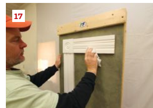
Scuffing the primer. Applying primer raises the grain on a wood surface, so light sanding is always required before finish coats. The author scuffs over every surface with fine-grit sand paper, taking care not to break through the painted surface (15). A small but powerful LED light helps him sight down all painted surfaces as he looks for areas that need to be sanded (16). When he is satisfied, he vacuums the entire trim area and finishes by wiping everything down with a damp rag (17).
