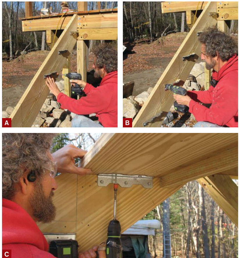
Figure 3. When installing the metal brackets, be sure to provide clearance for the structural riser (A). Before installing the treads, drill pilot holes for the structural screws that will be driven through the stringers and into the treads and risers (B). Structural screws are used to fasten the treads to the brackets (C).
