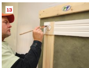
Priming. All coats of paint, including primer, should be brushed on in a deliberate sequence. The author begins at the top edge of the head casing (11), then brushes the bottom edge and the face (12). Next, he moves to the rosette, painting the edges first and then the face (13). Finally, he paints the vertical trim pieces (14). If this had been a complete casing, he would have finished with the sill and apron.
