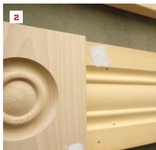
Filling holes. The author uses a flexible putty knife to fill the fastener holes with light- to medium-bodied filler (1). He leaves plenty of filler on the surface so that the filled hole can be sanded rather than filled a second time (2). In the grooved areas of the molding, he fills fastener holes with his little finger (3).
