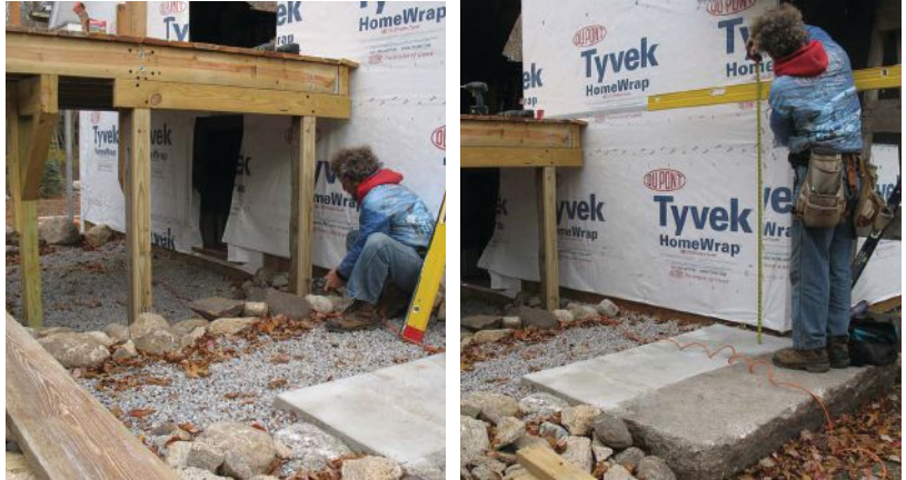
Figure 1. A dropped 2x6 header fastened to support posts provides a solid attachment point for the stairs (above left). Rise and run—and therefore the size of the risers and treads—is determined by marking a level line from the top of the decking, and then measuring out from the front edge of the decking and up from the end point of the stairs on the landing (above right).
