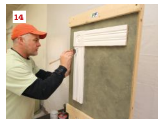
Priming. All coats of paint, including primer, should be brushed on in a deliberate sequence. The author begins at the top edge of the head casing (11), then brushes the bottom edge and the face (12). Next, he moves to the rosette, painting the edges first and then the face (13). Finally, he paints the vertical trim pieces (14). If this had been a complete casing, he would have finished with the sill and apron.
