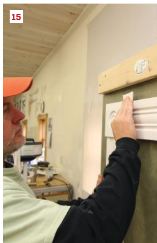
Scuffing the primer. Applying primer raises the grain on a wood surface, so light sanding is always required before finish coats. The author scuffs over every surface with fine-grit sand paper, taking care not to break through the painted surface (15). A small but powerful LED light helps him sight down all painted surfaces as he looks for areas that need to be sanded (16). When he is satisfied, he vacuums the entire trim area and finishes by wiping everything down with a damp rag (17).
