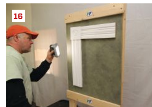
Priming. All coats of paint, including primer, should be brushed on in a deliberate sequence. The author begins at the top edge of the head casing (11), then brushes the bottom edge and the face (12). Next, he moves to the rosette, painting the edges first and then the face (13). Finally, he paints the vertical trim pieces (14). If this had been a complete casing, he would have finished with the sill and apron.
