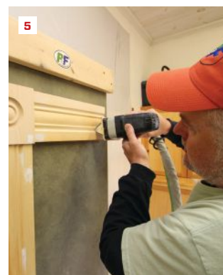
Power sanding. Sanding with machines allows the addition of a dust-collection system. Here, a sander with a flat sanding pad works on a filled hole (4). Linear profile sanders with different-shaped attachments work well on trim details such as grooves (5).
