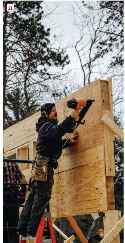
A load-bearing window wall. Carpenters Alex Strugatskiy and Will Kessler framed in the window opening between two large glulam carrying beams with 2x6 lumber. Strugatskiy laid out stud locations (9), boxed out the window opening (10), and then nailed plywood sheathing onto the face of the wall to stiffen the structure (11).
