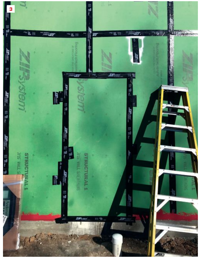
The Aarow Building crew leaves window and door openings (2) sheathed for the duration of the framing. When the frame is complete, they'll come back, fill in doors they left open for access (3), and run their initial blower-door test. Note the white spray paint above the door. All temporary nailers are painted white for easy identification so they can be filled prior to the test.
