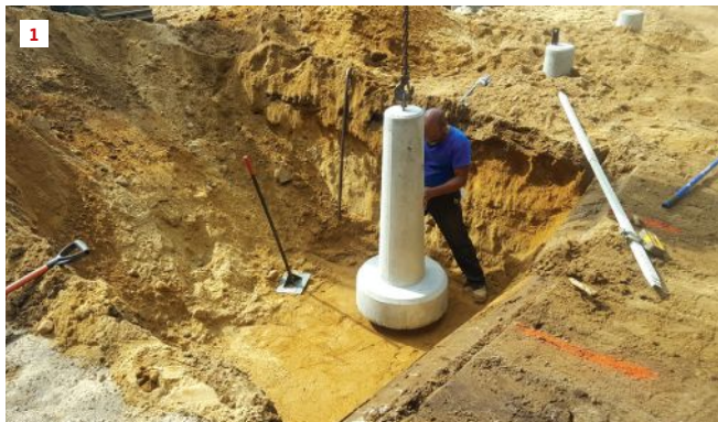
The site crew dug the hole for each precast footing individually, compacting the base of the hole and using a laser level to set the elevation (1). Each footing has an integral fitting for an eyebolt that was used to lift and place the footing (2). After the footings were placed, the crew used the fittings to attach the post connectors.
