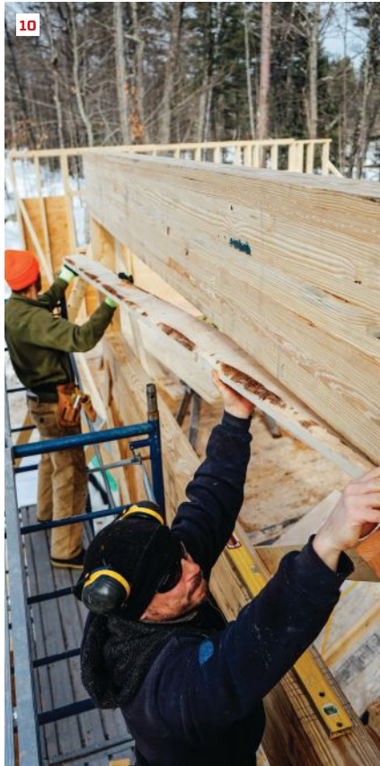
A load-bearing window wall. Carpenters Alex Strugatskiy and Will Kessler framed in the window opening between two large glulam carrying beams with 2x6 lumber. Strugatskiy laid out stud locations (9), boxed out the window opening (10), and then nailed plywood sheathing onto the face of the wall to stiffen the structure (11).
