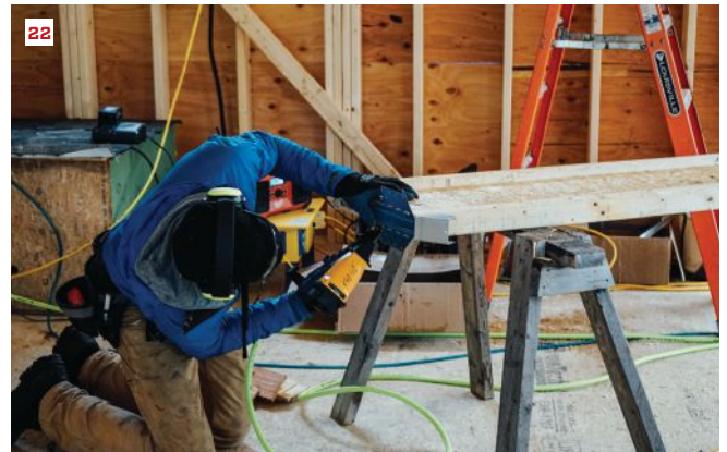
Prepping wood I-joint rafters. Jesper Kruse and carpenter Anna Heath made rafter plumb cuts using a site-built jig (19). Carpenter Ryan Bielenda packed out each rafter web with plywood stiffeners (20, 21) and then pre-applied Simpson adjustable wood I-joint hangers (22), which can be adjusted in the field to the necessary angle for a sloped or skewed connection.
