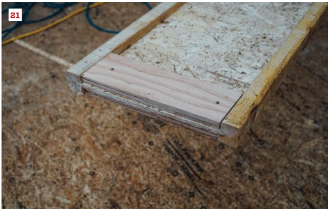
Prepping wood I-joint rafters. Jesper Kruse and carpenter Anna Heath made rafter plumb cuts using a site-built jig (19). Carpenter Ryan Bielenda packed out each rafter web with plywood stiffeners (20, 21) and then pre-applied Simpson adjustable wood I-joint hangers (22), which can be adjusted in the field to the necessary angle for a sloped or skewed connection.
