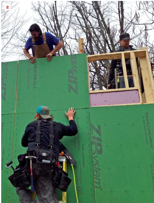
The Aarow Building crew leaves window and door openings (2) sheathed for the duration of the framing. When the frame is complete, they'll come back, fill in doors they left open for access (3), and run their initial blower-door test. Note the white spray paint above the door. All temporary nailers are painted white for easy identification so they can be filled prior to the test.
