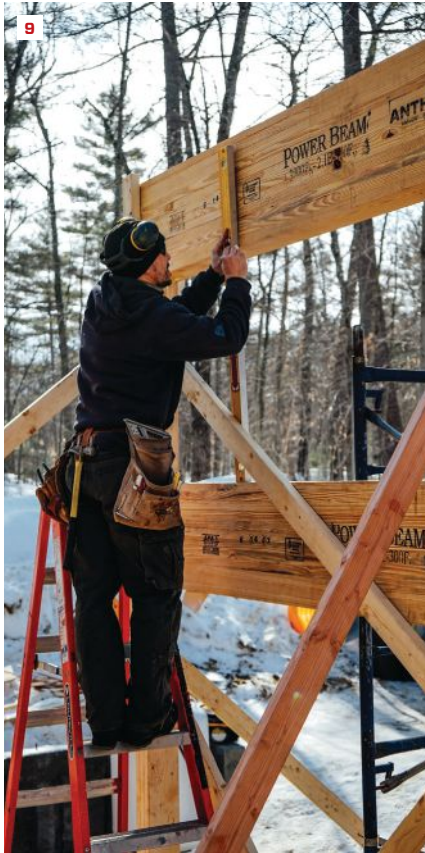
A load-bearing window wall. Carpenters Alex Strugatskiy and Will Kessler framed in the window opening between two large glulam carrying beams with 2x6 lumber. Strugatskiy laid out stud locations (9), boxed out the window opening (10), and then nailed plywood sheathing onto the face of the wall to stiffen the structure (11).
