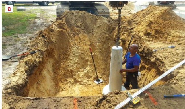
The site crew dug the hole for each precast footing individually, compacting the base of the hole and using a laser level to set the elevation (1). Each footing has an integral fitting for an eyebolt that was used to lift and place the footing (2). After the footings were placed, the crew used the fittings to attach the post connectors.
