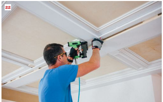
Nailing blocks fill in between the panels and the major-beam framing (19). A 2 1 / 2 -inch strip nails in along the major beams to create the intermediate layer (20). Pieces of pine 5 1 / 2 inches wide span between the panel sections for the minor beams (21). A crew member drives nails in the corner to keep the minor beams aligned with the 2 1 / 2 -inch strips (22).
