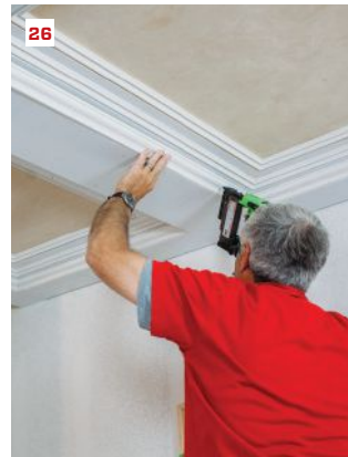
Panel molding transitions from the framed panels to the minor beam (23), while a bed molding transitions between the minor-beam and major-beam layers (24). To ensure that the reveal at the bottom of the bed molding stays consistent, the author scribes and planes problem areas (25) before nailing them into place (26). Panel molding dresses up the bottoms of the minor beams (27).
