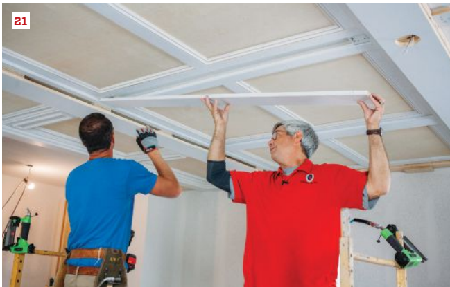
Nailing blocks fill in between the panels and the major-beam framing (19). A 2 1 / 2 -inch strip nails in along the major beams to create the intermediate layer (20). Pieces of pine 5 1 / 2 inches wide span between the panel sections for the minor beams (21). A crew member drives nails in the corner to keep the minor beams aligned with the 2 1 / 2 -inch strips (22).
