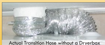
Actual Transition Hose without a Dryerbox
