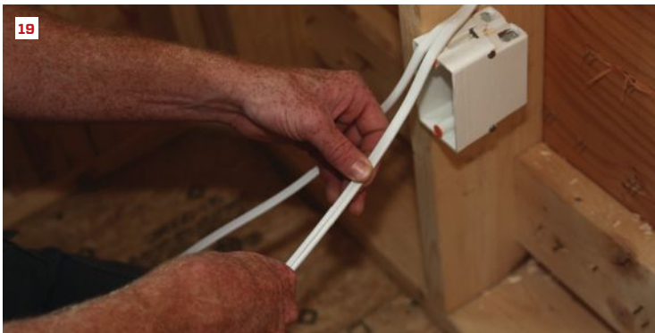
Receptacle box. The author's finger gauges where to strip off the outer jacket (18). A utility knife slits the jacket (19). (He adds an inch for slitting the second cable.) Looping cable into the box (20) provides extra cable in case of damage during drywalling.
