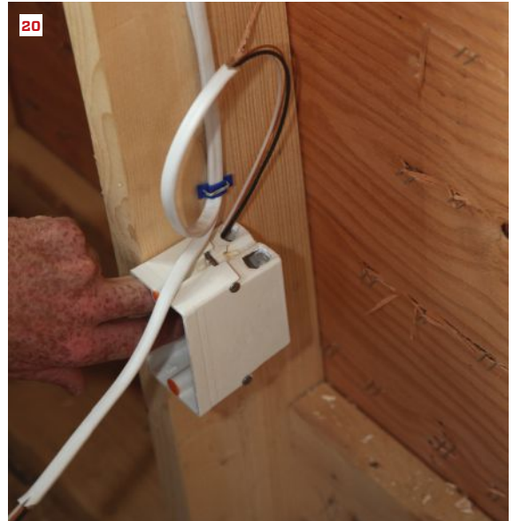
Receptacle box. The author's finger gauges where to strip off the outer jacket (18). A utility knife slits the jacket (19). (He adds an inch for slitting the second cable.) Looping cable into the box (20) provides extra cable in case of damage during drywalling.
