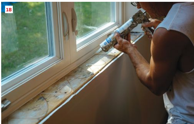
The author fills pinholes using a paste of cement, pozzolan, and acrylic fortifier (16) and applies ICT PS1 Reactive Sealer to the surfaces of the windowsills (17). On site, the installers apply a setting bed of silicone caulk to the rough framing (18), then set the concrete windowsills into place (19).
