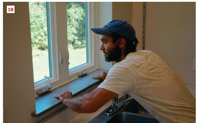
The author fills pinholes using a paste of cement, pozzolan, and acrylic fortifier (16) and applies ICT PS1 Reactive Sealer to the surfaces of the windowsills (17). On site, the installers apply a setting bed of silicone caulk to the rough framing (18), then set the concrete windowsills into place (19).
