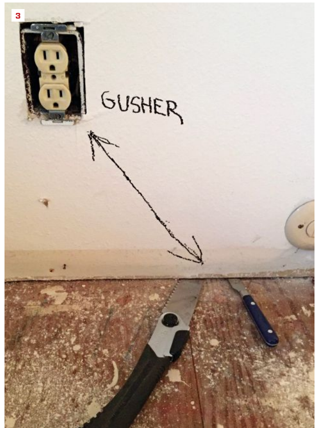
Working from the inside, the author probed with a strap tie to reveal the worst leaks in the house at the bottom plates (1) . At one place, where an exterior door was being replaced, the complete path of the air leaking into the wall cavity is revealed (2) . During an early blower-door test, the air flowing through this outlet and from the crack at the base of the wall gushed air (3) .
