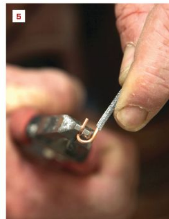
After rough-in, wires, or conductors, sit in the box, ready to be attached (1) . The author cuts the conductors, leaving the ground slightly longer (2) . Wire strippers remove an inch or so of insulation from each conductor (3) . To form a loop, grab the end of a conductor with pliers (4) and twist it into a U (5) , making sure the bare end is even with the end of the insulation.
