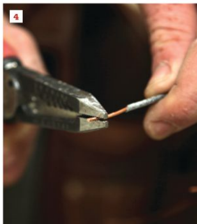
After rough-in, wires, or conductors, sit in the box, ready to be attached (1) . The author cuts the conductors, leaving the ground slightly longer (2) . Wire strippers remove an inch or so of insulation from each conductor (3) . To form a loop, grab the end of a conductor with pliers (4) and twist it into a U (5) , making sure the bare end is even with the end of the insulation.
