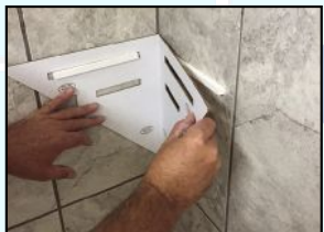
Glue on rails in slots
