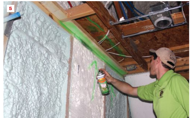
Technician Jack Hogan zeros the electronic manometer before the blower-door test (3). Hogan points out an air leak near the patio door (4). Hovis marks a gap in the foam insulation for correction by the foam crew (5).
