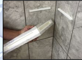
Silicone back and fill grooves
