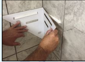
Glue on rails in slots
