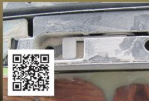
Window Sash Repair
