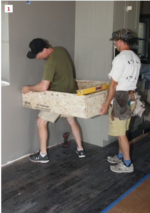
Jesper Kruse and carpenter Alex Strugaskiy screwed a plywood mock-up of the stair landing to the house wall (1) . Kruse leveled, squared, and braced the landing template (2) before measuring and cutting the stringers.
