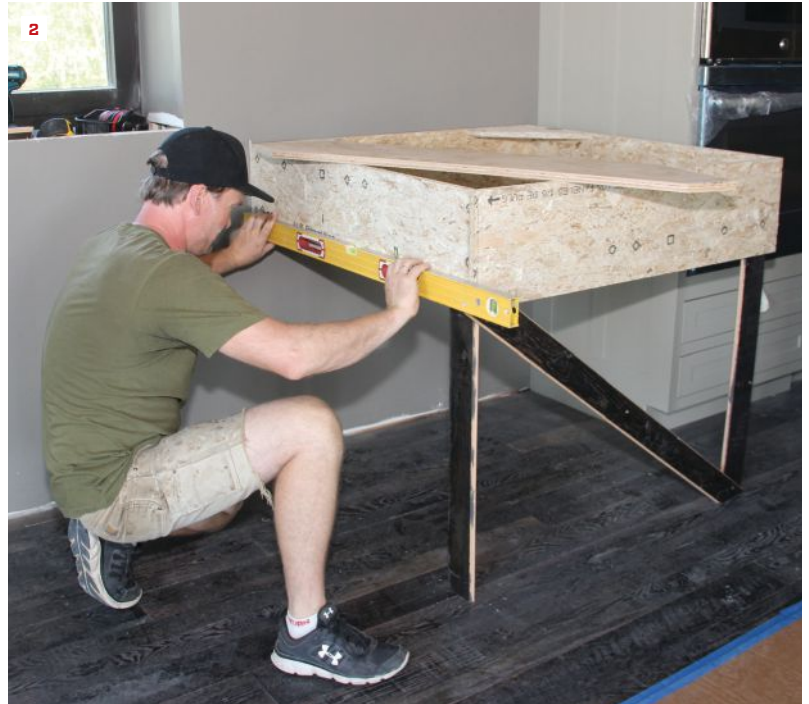
Jesper Kruse and carpenter Alex Strugaskiy screwed a plywood mock-up of the stair landing to the house wall (1) . Kruse leveled, squared, and braced the landing template (2) before measuring and cutting the stringers.
