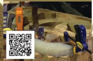
Decorative Corbel Repair
