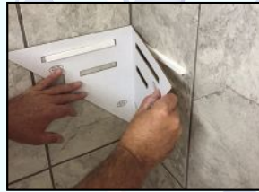
Glue on rails in slots
