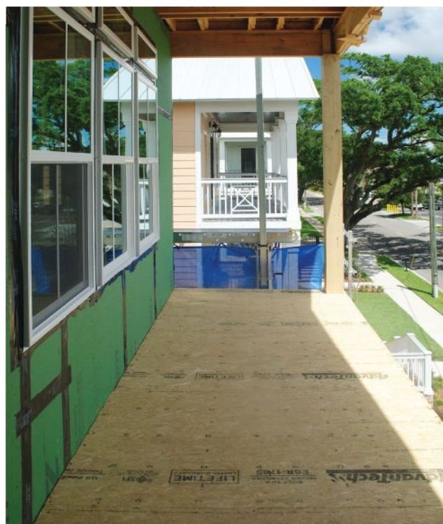
From top left: General Contractor John Price leads residential and light commercial projects for Gulfport, Mississippi-based Sapphire Homes. With many coastal projects, the company used ZIP System sheathing and tape for sealed roof decks and exterior walls to mitigate risk of water intrusion.
