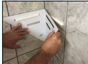
Glue on rails in slots
