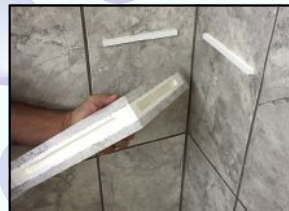
Silicone back and fill grooves
