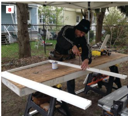
The author slides the door unit into place (5) and attaches the hinge jamb to his PVC blocks (6). Flashing tape seals the jambs to the foundation (7). An extension screws to the back of the exterior trim to accommodate the out-of-plumb foundation (8).
