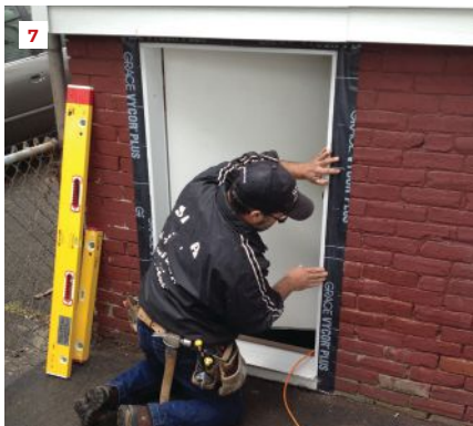
The author slides the door unit into place (5) and attaches the hinge jamb to his PVC blocks (6). Flashing tape seals the jambs to the foundation (7). An extension screws to the back of the exterior trim to accommodate the out-of-plumb foundation (8).
