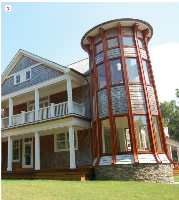
The paint-grade paneling on the first floor (1) and the mahogany paneling on the second floor (2) of this two-story tower (3) on Long Island, N.Y., were made with laminated stiles and rails and 1/4-inch plywood, using the same basic techniques. The plywood fits into a rabbet formed between the laminations in the stiles and rails.
