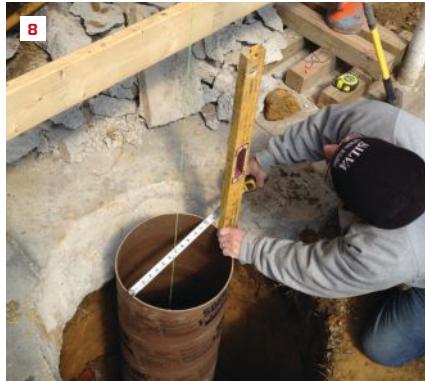
With the base cut to the right size, a cardboard form is screwed to it (5). The form height is measured from the beam above (6) and marked with a length of flashing tape (7). A measuring tape and level position the form precisely in the hole (8).
