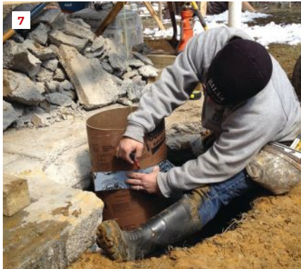
With the base cut to the right size, a cardboard form is screwed to it (5). The form height is measured from the beam above (6) and marked with a length of flashing tape (7). A measuring tape and level position the form precisely in the hole (8).
