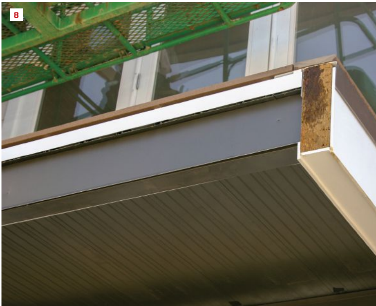
Wahoo Deck's Dry Joist EZ—a 2-inch-high aluminum joist system with an interlocking design—spans the distance between the LVL beams (7). The system can span up to 8 feet, depending on floor loads. Any standard decking can be attached to the aluminum joists; water that makes its way into the deck's interior drains to the outer edge (8).
