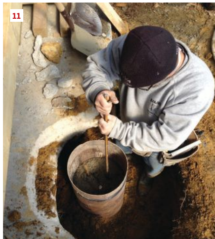
A backfill layer keeps the form in place for the pour (9). The form is pumped dry and concrete is placed (10). When the concrete is near the top of the form, three pieces of rebar are added to strengthen each footing (11). After the form is filled and the hole backfilled, the top of the footing is brushed even (12).
