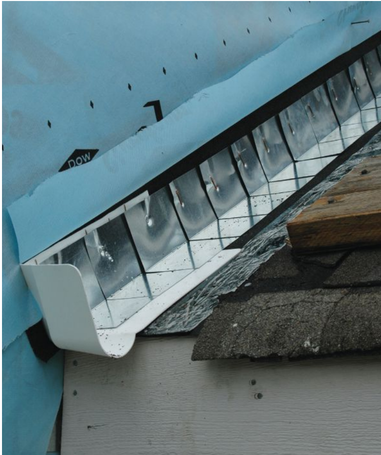
A pre-made, one-piece TPO kickout, like this one from DryFlekt, is large enough to deflect roof runoff into the (yet-to-be-installed) gutter.
