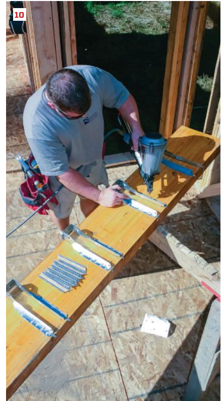
Shown above are two preassembly tricks that save time: A framer preattaches a rim joist to a girder before it is lifted into place with the forklift (9). On ledgers and rims, it also saves time to preinstall joist hangers (10). It's much easier and faster to do this on sawhorses than while balancing at the top of a ladder.
