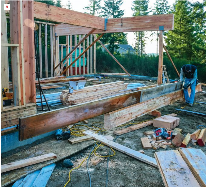
Shown above are two preassembly tricks that save time: A framer preattaches a rim joist to a girder before it is lifted into place with the forklift (9). On ledgers and rims, it also saves time to preinstall joist hangers (10). It's much easier and faster to do this on sawhorses than while balancing at the top of a ladder.
