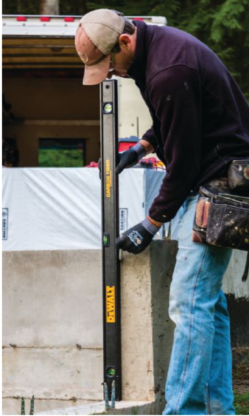
The DWHT43134 has two vials for plumb and one for level, two small hang holes, and small end caps that let you draw a line almost to the end of the level.
