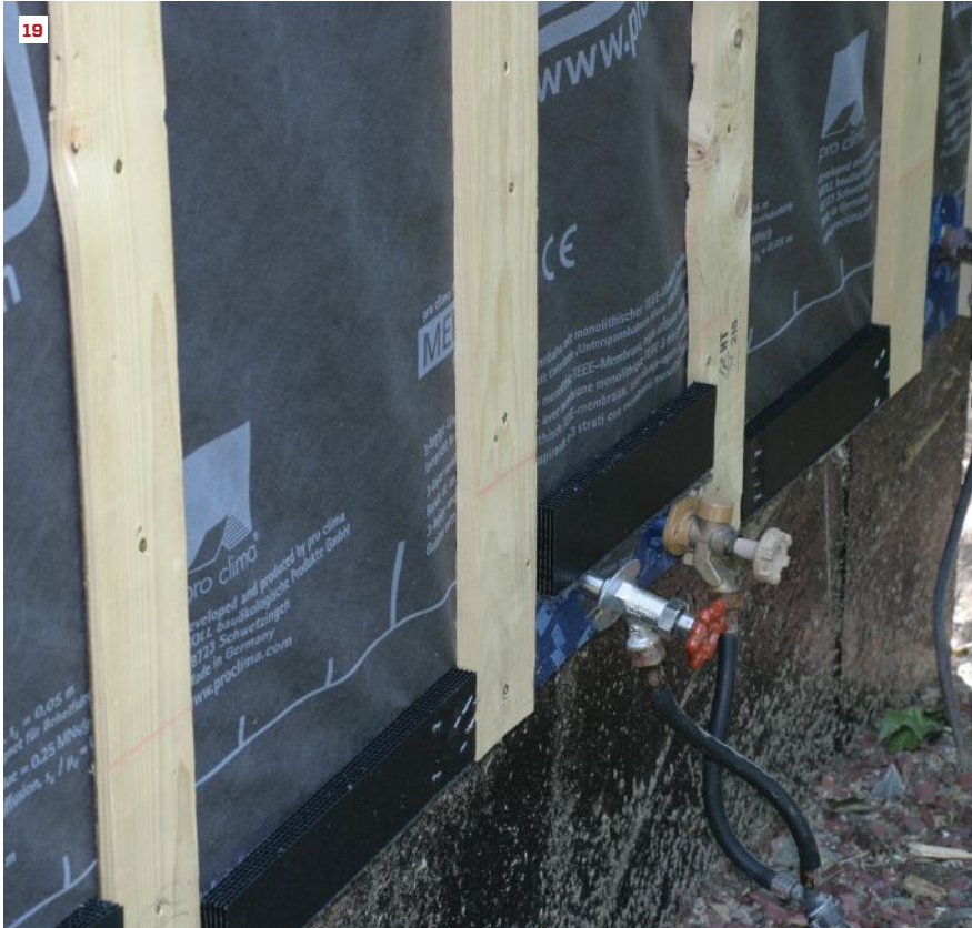
The crew installed insect-screening vent baffles at the base of wall between strapping pieces (19), then applied rot-proof, bug-proof Boral synthetic trim board to the wall (20, 21). Later, they would side the wall with HardiePlank fiber-cement lap siding.
