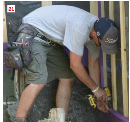
The crew installed insect-screening vent baffles at the base of wall between strapping pieces (19), then applied rot-proof, bug-proof Boral synthetic trim board to the wall (20, 21). Later, they would side the wall with HardiePlank fiber-cement lap siding.
