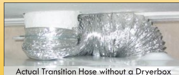
Actual Transition Hose without a Dryerbox
