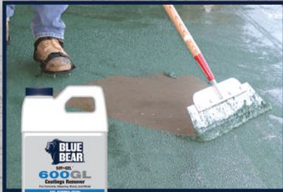
Removal of Floor Paint
