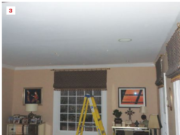
3. We knew some of this ceiling was wet from a bath leak above. But where exactly were the wet areas? 4. With the infrared camera, we could see the wet areas as cold spots (darker colors), showing the extent of the leak.
