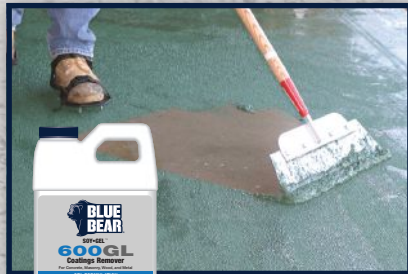
Removal of Floor Paint
