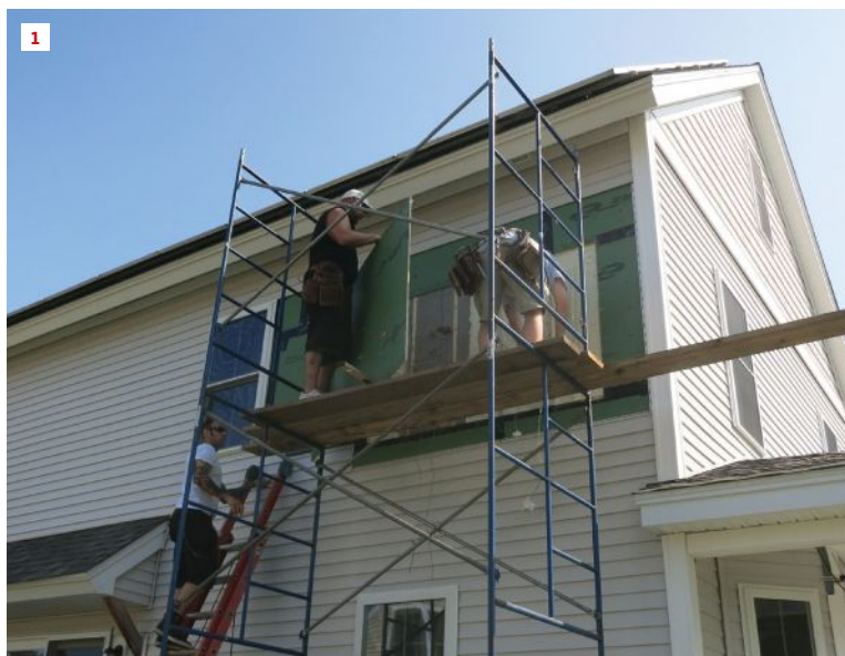
1. After three seasons of moisture and temperature monitoring, workers pull sections of Zip sheathing panels from the test wall section of a house in Devens, Mass.
