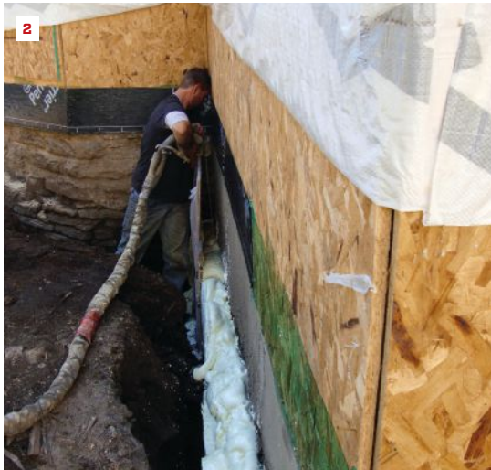
At wide spots in the trench, the foam is poured to a consistent thickness against a sheet of OSB.
