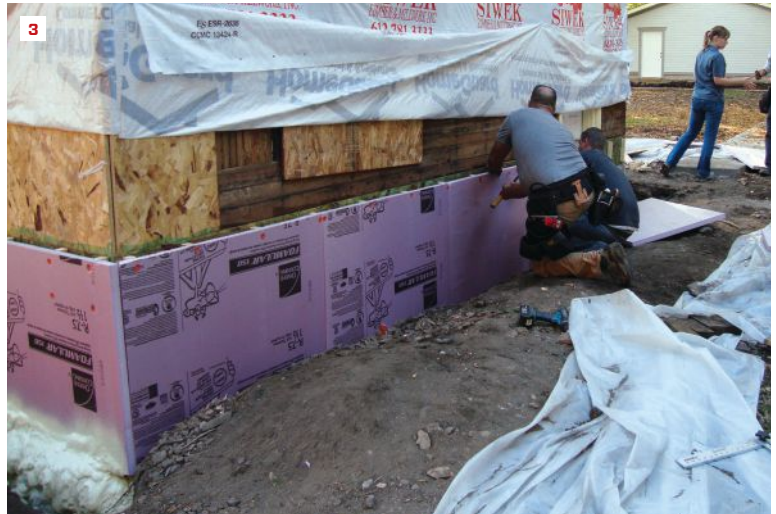
Rigid foam covers the rim joist. The top edge will be capped and flashed, and the face covered with an elastomeric parge coat.
