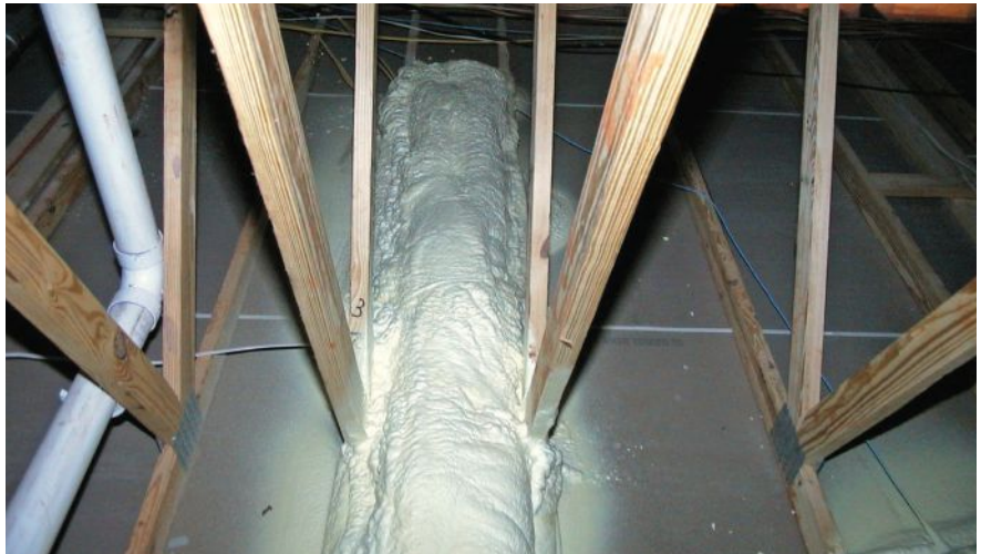
Duct encapsulation. Top: before drywall; bottom: after drywall.
