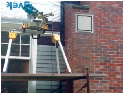
The lightweight saw can easily be set up on staging so it's close to the work.
