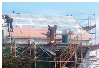
Figure 3. Plywood sheathing, screwed through the foam insulation on the roof and into the rafters, provided continuous nailing for the red cedar roof shingles. The seams were taped per the manufacturer's instructions, and a mesh drainage layer went between the sheathing and the shingles.
