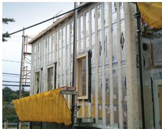
Figure 2. Before the nailing strips went on, cellulose insulation was blown into the walls; housewrap was attached to the original sheathing (above) to keep the cellulose from leaking out. Then the walls were wrapped with foil-faced foam and the seams taped. Vertical strapping was screwed through the foam and into the framing to attach the siding and trim (left). Extra stock was later added around window and door openings for nailers. Vent strips were installed at the top and bottom of each wall for drainage and to allow air to flow freely behind the clapboards (bottom).
