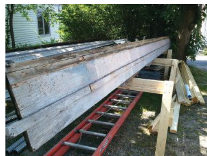
Figure 1. Before the renovation, the building was essentially sound, but the years had not been kind to it. Asbestos shingles covered the walls (left), and much of the trim had deteriorated beyond saving. As the exterior layers were peeled back, any of the original cypress trim that still had life was set aside to be reinstalled later (above).
