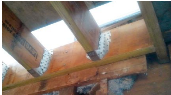
Figure 4. When the trim went back on the building, original detailing was followed as closely as possible based on archival photos and the trim that was removed (above). Metal connectors and beams were added where the old structure needed strengthening (left).
