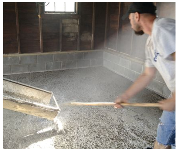
Figure 8. After laying down a layer of 4-inch gravel, reinforced 6-mil poly sheeting, and welded-wire mesh, the crew ran asphalt-impregnated fiberboard around the inside face of the footing (left), then poured the new 4-inch slab flush with the top of the footing (right). The fiberboard serves to isolate the slab from the footing should any frost issues arise.
