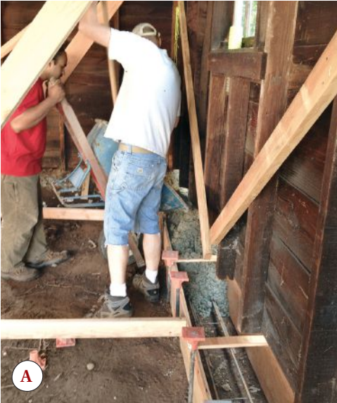
Figure 3. The bracing strategy was designed to support one wall at a time (left). To avoid damage to the existing shell, squaring up and leveling was kept to a minimum. New 14-inch-deep footing forms were set at the same height as the existing slab and tied back to the diagonal bracing (right).
