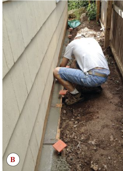
Figure 3. The bracing strategy was designed to support one wall at a time (left). To avoid damage to the existing shell, squaring up and leveling was kept to a minimum. New 14-inch-deep footing forms were set at the same height as the existing slab and tied back to the diagonal bracing (right).
