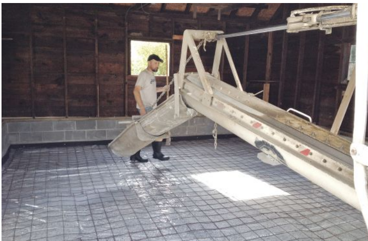
Figure 8. After laying down a layer of 4-inch gravel, reinforced 6-mil poly sheeting, and welded-wire mesh, the crew ran asphalt-impregnated fiberboard around the inside face of the footing (left), then poured the new 4-inch slab flush with the top of the footing (right). The fiberboard serves to isolate the slab from the footing should any frost issues arise.
