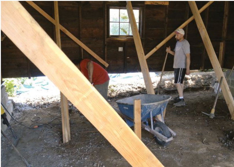
Figure 5. With the gable-end walls done, the existing rear wall could be readied for formwork (above). Similar to the gable-end footings, two continuous #5 rebars were placed at the bottom of the footing (right). The rear footing was pinned to the gable ends with two #5 rebar pins drilled and epoxied into place.
