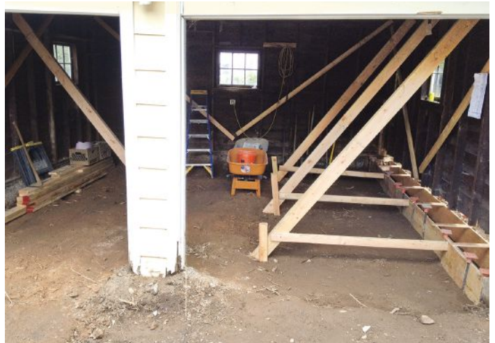
Figure 3. The bracing strategy was designed to support one wall at a time (left). To avoid damage to the existing shell, squaring up and leveling was kept to a minimum. New 14-inch-deep footing forms were set at the same height as the existing slab and tied back to the diagonal bracing (right).
