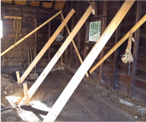
Figure 3. The bracing strategy was designed to support one wall at a time (left). To avoid damage to the existing shell, squaring up and leveling was kept to a minimum. New 14-inch-deep footing forms were set at the same height as the existing slab and tied back to the diagonal bracing (right).
