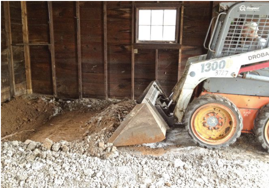
Figure 2. When the author's crew demoed the garage's existing 2-inch-thick slab (above), they discovered that the walls were bearing on cinder blocks placed on their side, with the existing slab keyed into the voids. Even with this thickened edge, the sill plates were 90% gone, due to their proximity to grade (right).
