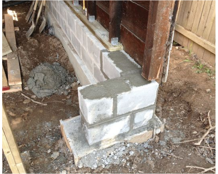
Figure 6. Like the rear footing, the front wall footing returns are pinned to the new gable-end footings with two #5 rebars (above), and the blocks were toothed together at the corner (right).
