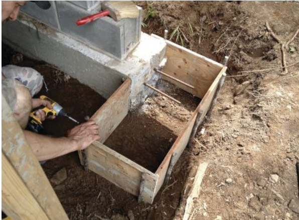
Figure 6. Like the rear footing, the front wall footing returns are pinned to the new gable-end footings with two #5 rebars (above), and the blocks were toothed together at the corner (right).
