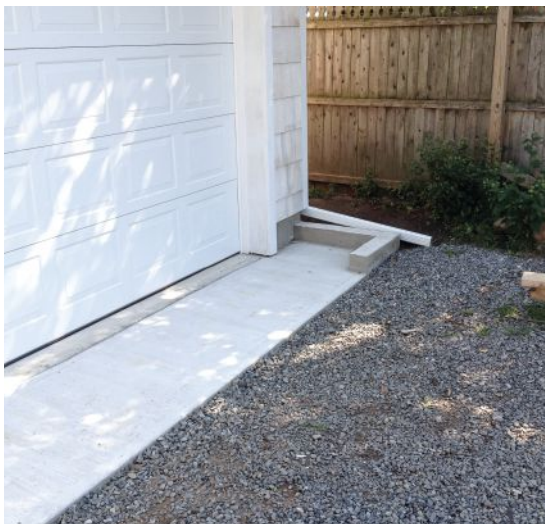
Figure 10. The bulk of the exterior finishes are on the front wall; new siding flanks a car-and-a-half-wide garage door (above). The exposed block stem wall was parged with mortar, and the driveway was regraded with new gravel. Gutters were added, and a berm was created to help direct runoff away from the entry apron (left).
