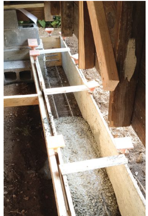
Figure 5. With the gable-end walls done, the existing rear wall could be readied for formwork (above). Similar to the gable-end footings, two continuous #5 rebars were placed at the bottom of the footing (right). The rear footing was pinned to the gable ends with two #5 rebar pins drilled and epoxied into place.
