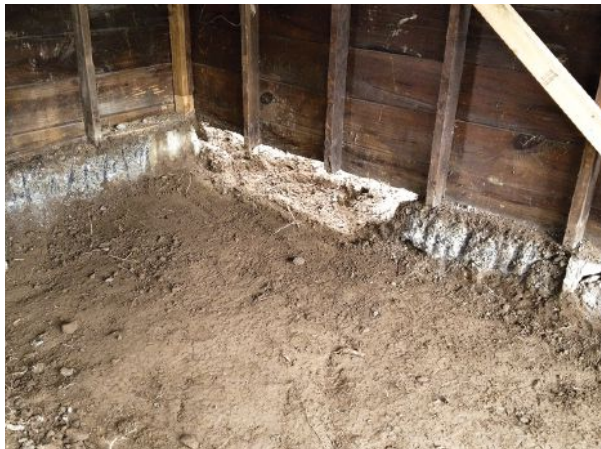
Figure 2. When the author's crew demoed the garage's existing 2-inch-thick slab (above), they discovered that the walls were bearing on cinder blocks placed on their side, with the existing slab keyed into the voids. Even with this thickened edge, the sill plates were 90% gone, due to their proximity to grade (right).
