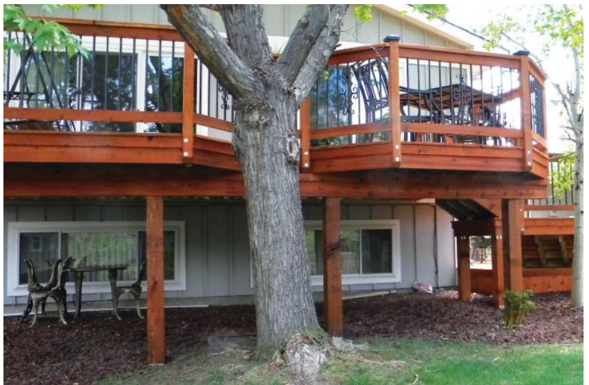
Figure 12. Support columns and railing posts made from wood (left) are simpler and cheaper than ones of steel. Once everything is wrapped with finish materials, it's impossible to tell what the underlying material is (below).
