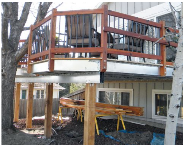
Figure 12. Support columns and railing posts made from wood (left) are simpler and cheaper than ones of steel. Once everything is wrapped with finish materials, it's impossible to tell what the underlying material is (below).
