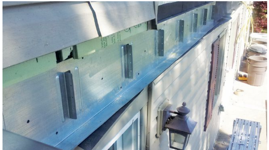
Figure 6. Ledger and rim track is available with tabs punched on standard framing layouts (above). The joists are screwed to these tabs (left).
