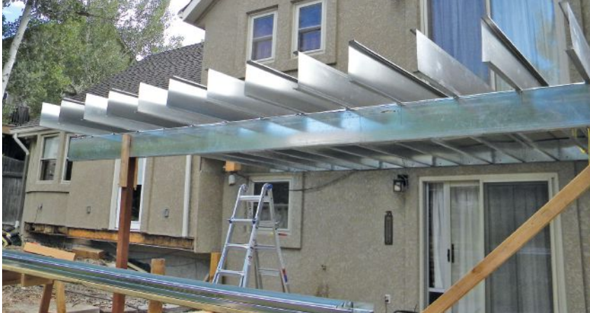
Figure 3. Although steel can span considerably longer distances than wood, it's only about one-third the weight.
