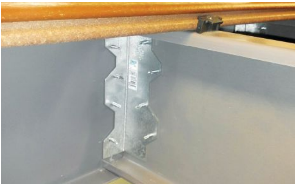
Figure 5. Some steel framing systems require the use of framing hardware to make connections.
