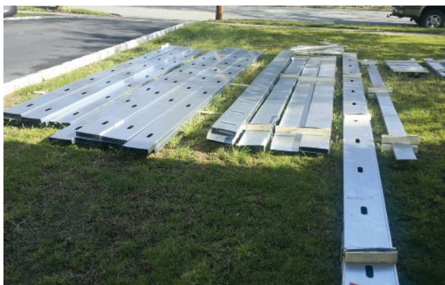
Figure 2. The author buys steel framing members pre-cut to the exact length needed.
