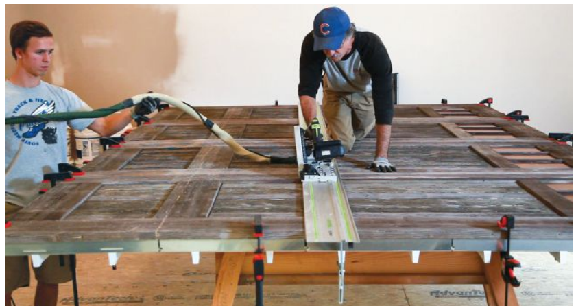
Figure 6. The author cut through the carriage doors using a track-mounted saw for accuracy (above). The blade was set with a slight 2-degree bevel for drainage (left).
