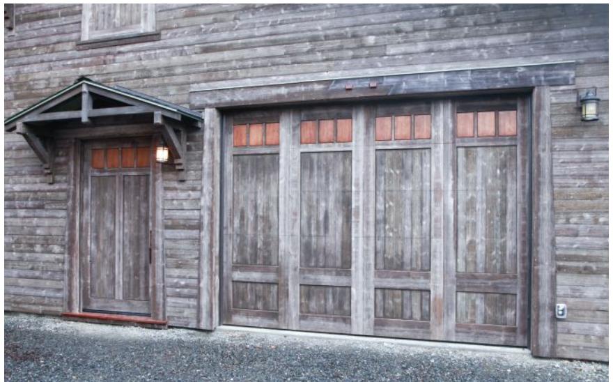
Figure 7. The door company used special track-mounting hardware to accommodate the 3 1 / 4 -inch-thick door (above). Each of the five roll-up panels weighs 120 pounds (above right), but the assembled door (right) is easily operated by one person, thanks to the commercial-style coil spring counterweight mechanism.
