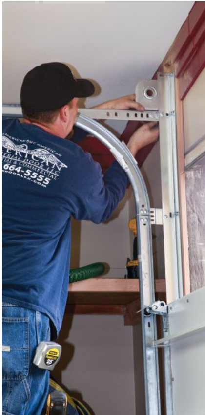
Figure 7. The door company used special track-mounting hardware to accommodate the 3 1 / 4 -inch-thick door (above). Each of the five roll-up panels weighs 120 pounds (above right), but the assembled door (right) is easily operated by one person, thanks to the commercial-style coil spring counterweight mechanism.
