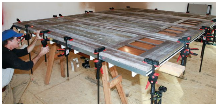
Figure 5. Once the carriage doors were assembled, the author spread construction adhesive on the steel door panels (left), then clamped the carriage doors in place (below). Dozens of 3-inch self-tapping coated screws driven through the backs of the roll-up panels into the stiles and rails of the carriage doors join the wood and steel door sections together.
