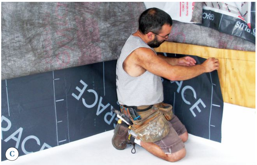
Figure 4. Because seams at inside corners leave a potential pinhole leak where the deck and walls intersect, a prefabricated corner piece is heat-welded to all three surfaces (A, B). Peel-and-stick membrane flashing adhered to the sheathing (C) will later be covered with housewrap.
