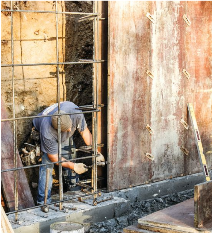
Figure 4. The author forms 8-foot-tall walls vertically, placing snap ties in slots located 1, 2, 4, 6, and 7 feet along the panel edges.
