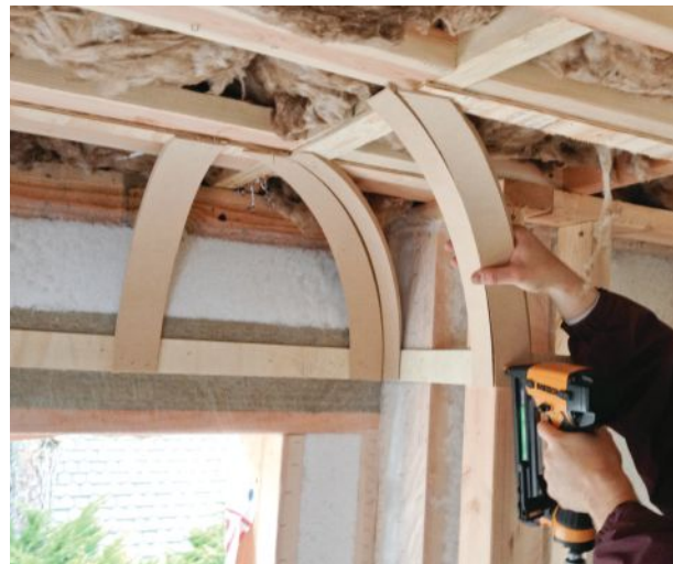
Figure 5. Inside and outside corner arches were also included in the kit. Pairs were butted together to form each corner and fastened in place with glue and staples.
