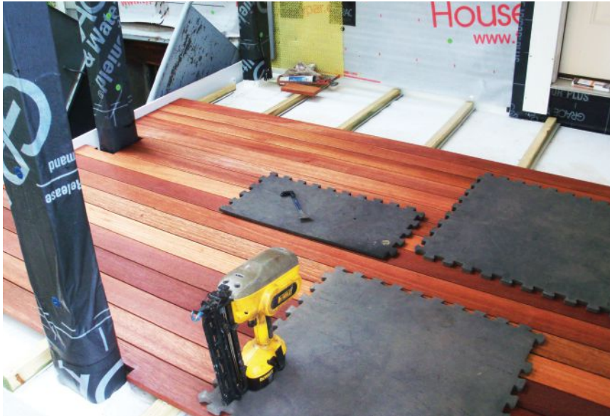
Figure 6. Once the completed membrane had been flashed and leak-tested, mahogany decking was fastened to tapered pressure-treated sleepers (left). The finished porch was trimmed out with PVC post and column wraps, moldings, and balusters, combined with mahogany stair treads, fascia trim, and railings (below).
