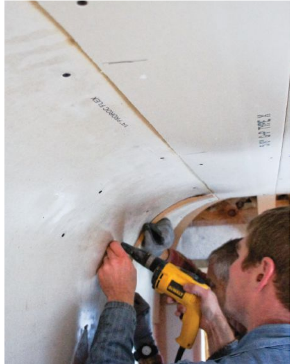
Figure 7. When forming the panels, crewmembers worked slowly and avoided pushing hard on the center of the panel, which would break the paper face and buckle the drywall (above). Once the panels conformed to the cove, they were screwed in place with regular drywall fasteners on 5-inch centers (right).
