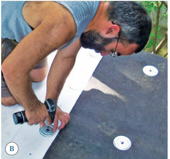
Figure 3. Cutouts in the membrane (A) allowed it to slip over the tops of the posts, minimizing seams; an open cutout at the outside corner column accommodates the membrane turn-down along both edges. The upper edge of the first sheet of membrane is screwed to the deck at 12-inch intervals. A preprinted line 4 inches from the edge marks the correct overlap for the next sheet (B). Turned-down membrane edges are secured to the PVC fascia with double-sided tape approved by the TPO manufacturer (C).
