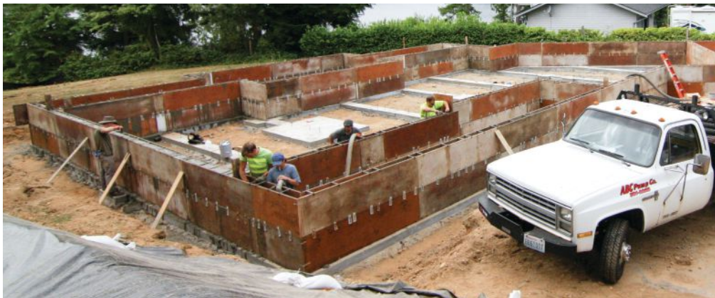
Figure 3. To build 4-foot or 6-foot-tall foundation walls, the author stacks his forms horizontally on snap ties laid across each lower course. Aligning the stacked panel joints vertically speeds installation and makes it easier to strip the forms later.
