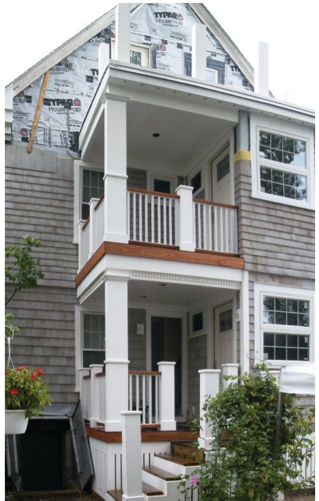
Figure 6. Once the completed membrane had been flashed and leak-tested, mahogany decking was fastened to tapered pressure-treated sleepers (left). The finished porch was trimmed out with PVC post and column wraps, moldings, and balusters, combined with mahogany stair treads, fascia trim, and railings (below).
