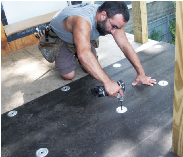
Figure 2. To protect against fastener show-through, the author added a layer of wood-fiber recover board, fastened to the structural deck with the same reinforced galvanized screw plates and 1 5 / 8 -inch screws used to secure the TPO membrane.
