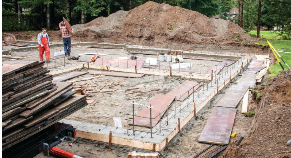
Figure 1. Workers finished up the steelwork before scattering the heavy Ply-form panels, with one continuous row of horizontal rebar about 3 inches up and another row at the top of the verticals.
