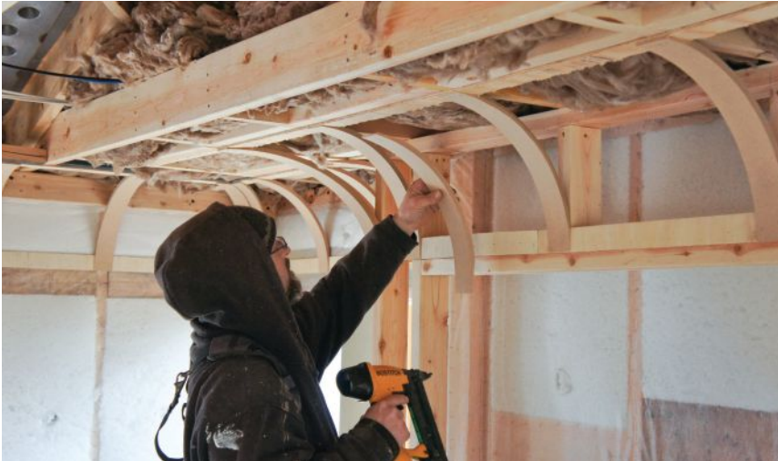
Figure 4. The arches were fastened to the furring strips 16 inches on-center. A narrow crown stapler and dabs of construction adhesive were used to make the attachment.
