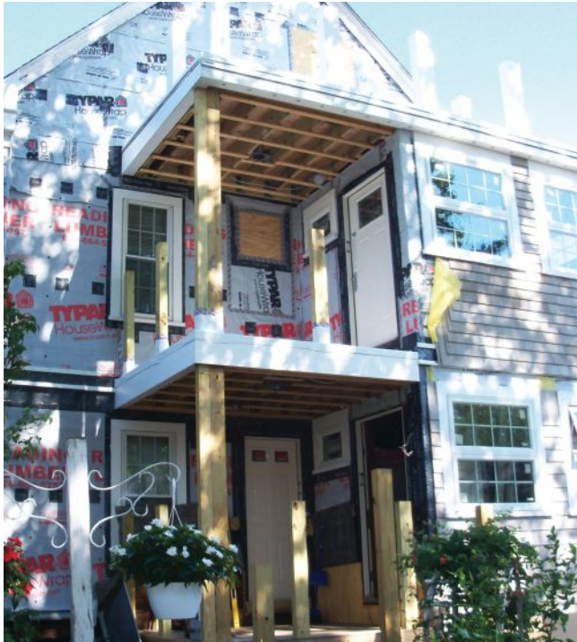
Figure 1. Using a membrane on all three decks ensures that water from rain or snowmelt will drain away from the house. On the ground-floor deck, the membrane keeps water away from the foundation, protects the underlying framing and connections, and allows for dry storage underneath.
