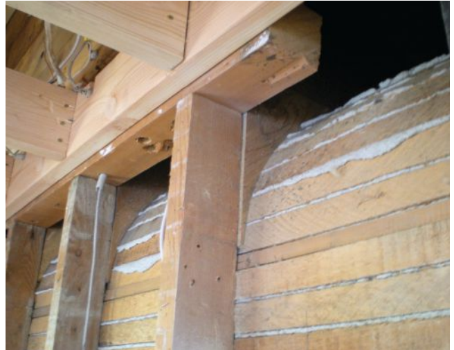
Figure 1. The ceilings in the original house had an interesting cove detail (above) that the homeowners wanted to duplicate in their new addition, but with typical drywall instead of traditional plaster-and-lath construction (right).
