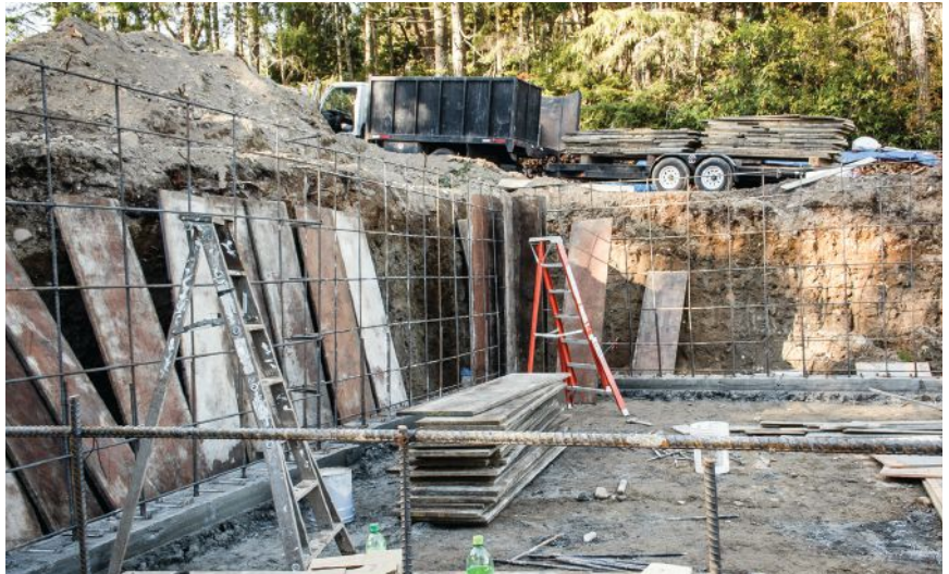
Figure 2. Reinforcement schedules for tall walls typically call for horizontal rebar on 12-inch to 18-inch centers depending on site conditions and structural requirements.
