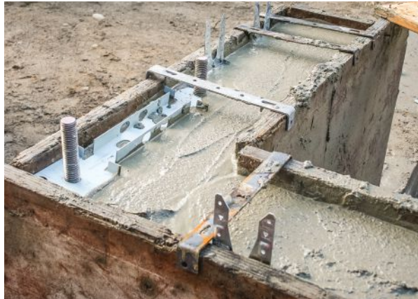
Figure 7. The author prefers Simpson MASA mudsill anchors over traditional anchor bolts for fastening the framing to the foundation. In the rush of the pour, this shear brace template was installed upside-down, so the author will just pop it out after the concrete has set up.
