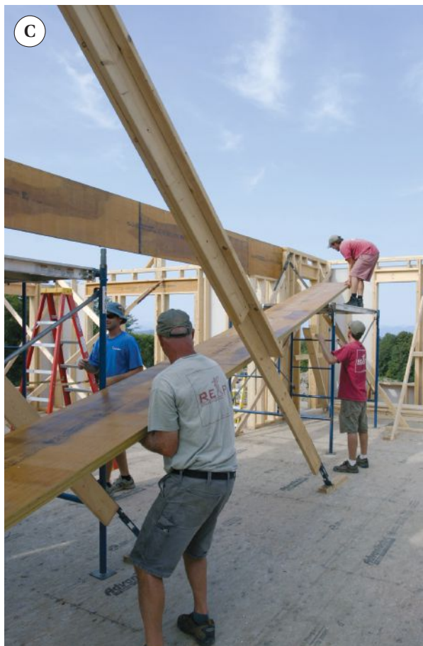
Figure 4. Once the first-floor walls were in place, the crew could install the second-floor support beams (A). While many of the beams were precut (B), a large 5 1 / 4 -inch-wide by 24-inch-deep by 28-foot-long beam built up from three 1 3 / 4 -inch by 24-inch LVLs was not, which allowed the crew to verify the length of the span, then cut and fit the beam one ply at a time (C).
