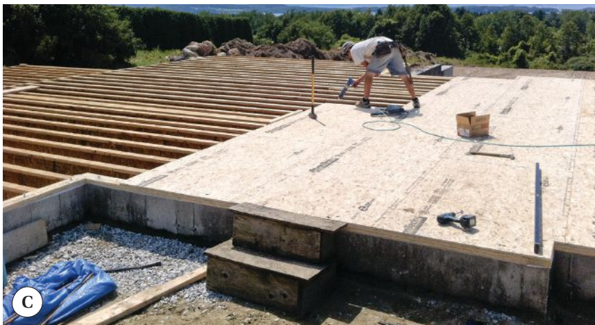
Figure 3. The LVL beams that support the first-floor framing are included in the JobPack package, along with supporting columns, metal connectors, and even the dimensional lumber used to frame the supporting walls (A). Joist layout is premarked on the LVL beams and LSL rim joists (B), which streamlines joist installation and allows the crew to quickly get the deck sheathed (C).
