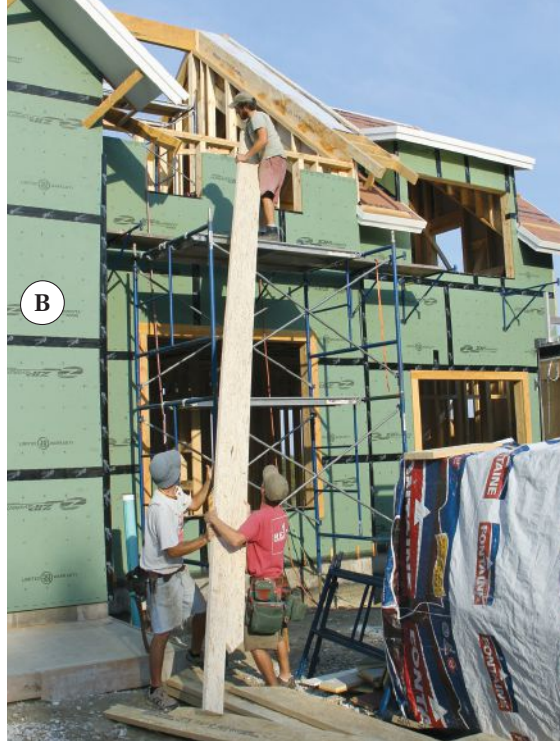
Figure 7. Some of the common rafters had to be cut on site from stock material (A). LSLs are a lot heavier than I-joists or sawn lumber; wrestling the 20-foot-long common rafters into position was a three-man job (B). Crew members tacked the dense material in place with a nail gun (C), then used impact drivers to drive structural screws through the rafters into the framing.
