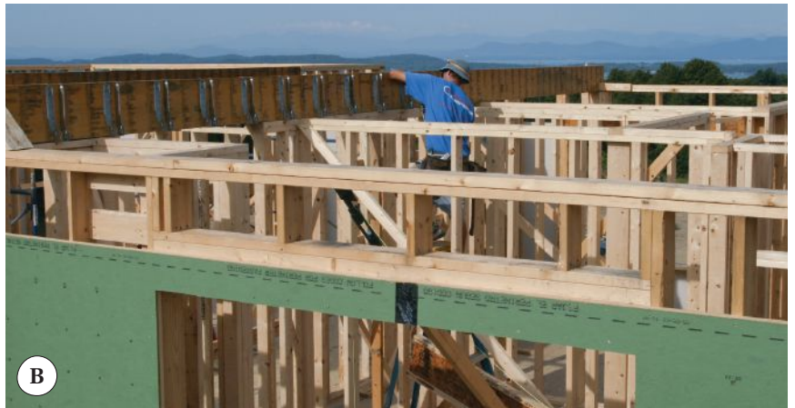
Figure 4. Once the first-floor walls were in place, the crew could install the second-floor support beams (A). While many of the beams were precut (B), a large 5 1 / 4 -inch-wide by 24-inch-deep by 28-foot-long beam built up from three 1 3 / 4 -inch by 24-inch LVLs was not, which allowed the crew to verify the length of the span, then cut and fit the beam one ply at a time (C).
