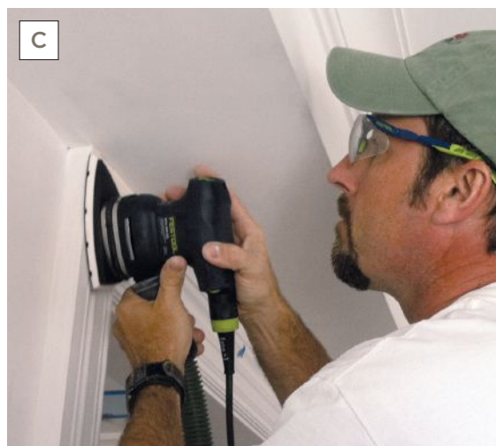
Figure 2. After patching nail holes and dings and sanding again, the author primes the trim (A) with a fast-drying sandable waterborne primer (B). Waterborne primers raise the grain, so once the primer has dried, he sands it with 150- to 180-grit paper to smooth out the surface and prepare it for top-coating (C).
