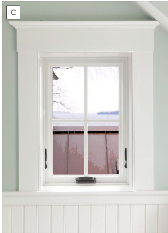
Figure 6. Waterborne trim paints tack up in less than an hour, reducing the risk of dust contamination (A). When properly applied, they produce a smooth cabinet-grade finish with a satin sheen (B, C).
