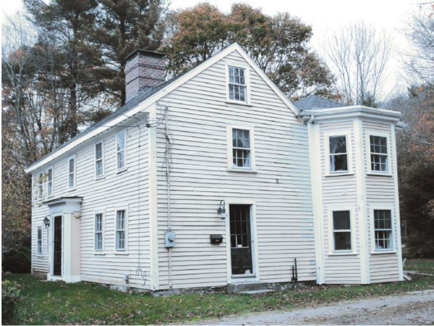
Figure 1. Though still intact after nearly 300 years, the framing of the gable roof needed reinforcement to eliminate a long-term sag of the roof deck between the widely spaced rafters.
