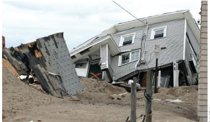
Along the Connecticut shore, the storm surge on the Long Island Sound destroyed shorefront houses.
