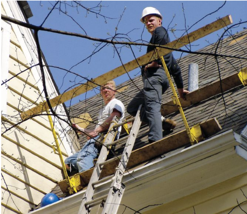
Figure 4. Roof jacks fitted with integral guardrails can be used instead of safety harnesses in certain situations, such as for flashing and repair work.
