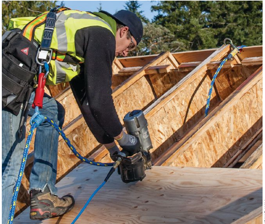
Figure 2. Anchors need to be strong enough to support 5,000-pound loads, so they must be securely fastened to framing.
