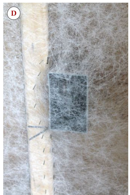
Figure 2. To minimize bulging of the cellulose between framing members, netting is stretched tight and fastened with a pneumatic upholstery stapler (A, B). The closely spaced fasteners are driven at an angle just beyond the outer edges of the faces of framing members. This “inset stapling” helps draw the material taut and prevents the cellulose from pushing beyond the framing (C). The tension of the netting against electrical boxes is enough to prevent them from filling with insulation when the cavities are packed; the netting will later be cut by the drywall crew (D).
