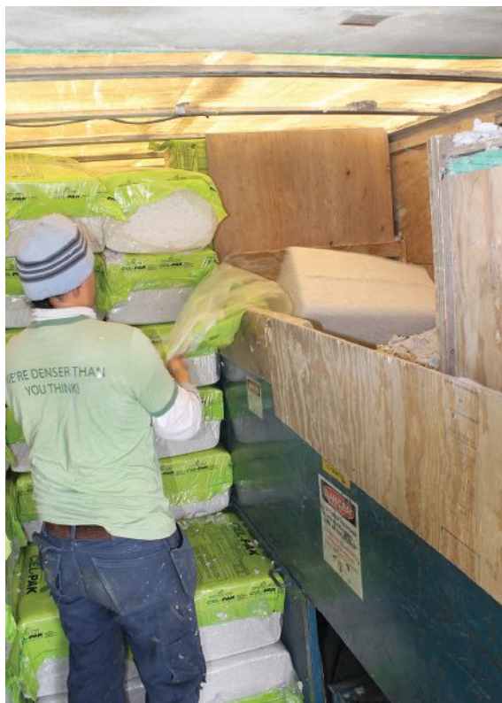
Figure 1. This truck (above) is equipped to install either damp-spray or dense-pack cellulose. The hopper that feeds material to the operator can be filled to the ceiling (right), providing enough material to last from 15 minutes to an hour, depending on the application.
