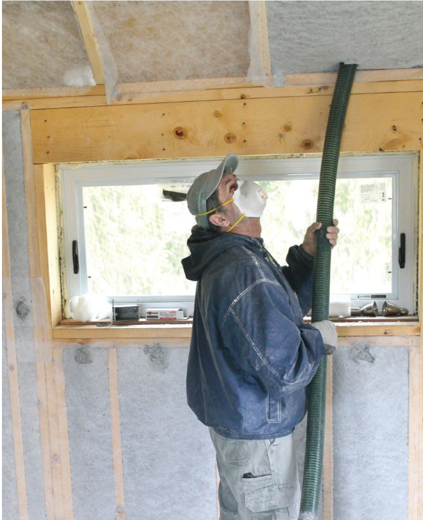
Figure 6. When filling rafter cavities, the usual insertion point is just above the top plate (above). The natural curvature of the longer hose required tends to direct the flow of insulation to one side of the cavity, so filling it uniformly requires a second pass with the curve facing the other way. The hose is visible behind the netting in the photo at right.
