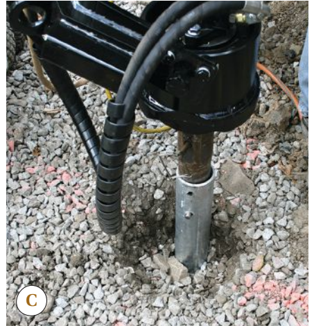
Figure 3. Shaft extensions are welded on and the pier driven as deep as needed to reach soil with adequate bearing capacity (A). The pier can be steered around a below-grade rock by moving the driver's boom; once the obstruction is passed, the boom pulls the shaft plumb again (B). Even though this pier penetrates about 13 feet into the ground, there's no pile of excavated soil as there would be with a conventional footing (C).
