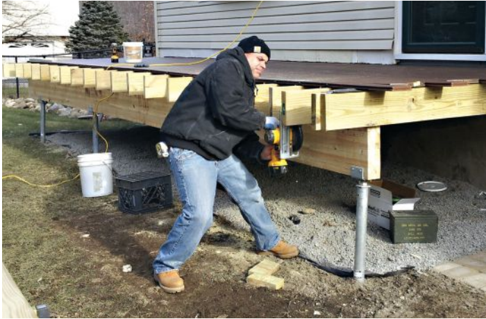
Figure 4. Above is a typical deck foundation using helical piers, which have greater bearing capacity than concrete piers and install with little disturbance to the landscape. At right, treated posts supporting a porch have been fastened to connector caps on the helical piers.
