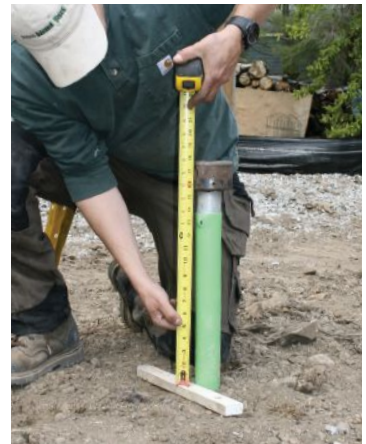
Figure 3. Shaft extensions are welded on and the pier driven as deep as needed to reach soil with adequate bearing capacity (A). The pier can be steered around a below-grade rock by moving the driver's boom; once the obstruction is passed, the boom pulls the shaft plumb again (B). Even though this pier penetrates about 13 feet into the ground, there's no pile of excavated soil as there would be with a conventional footing (C).
