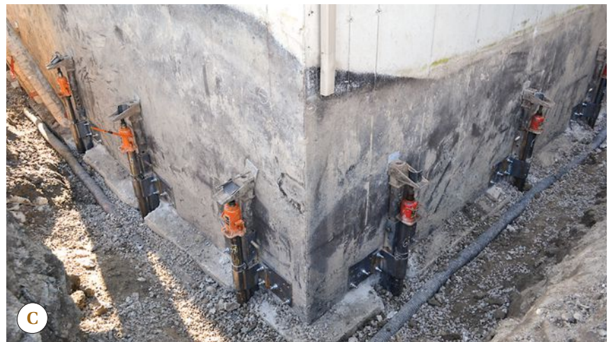
Figure 5. Adding a vertical extension to the drilling rig makes it possible to drive piers into steeply sloped sites (A). The machine is also well-suited to foundation stabilization work, as it can fit in tight spaces around existing homes (B). Piers are typically installed every 6 feet along an underpinned foundation (C).
