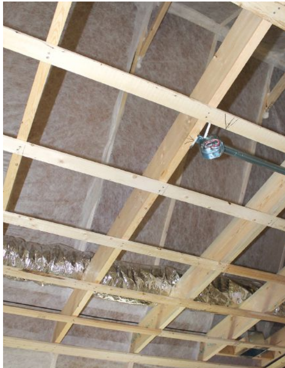
Figure 3. A skilled installer can snugly fit the netting around joists, collar ties, and other obstructions. As long as the material is tight and securely stapled, small gaps won't leak significant amounts of insulation as the cavities are blown full (right). In complex areas, like the peak of this Queen Anne tower (below), netted dense-pack can be a cost-effective alternative to spray foam.
