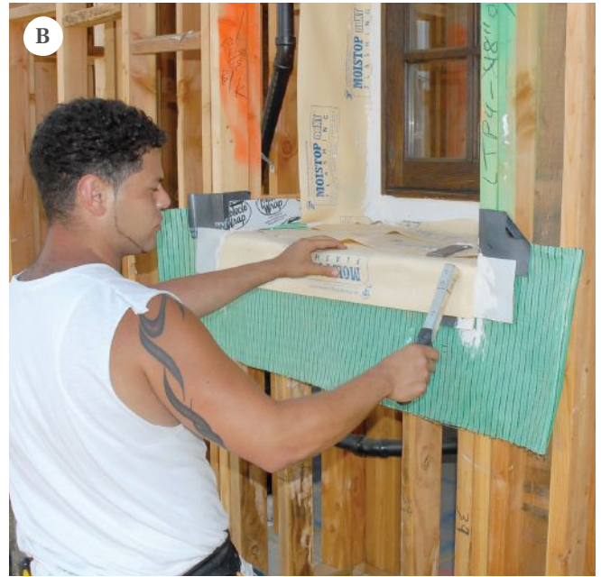
Figure 3. Prefabricated plastic corners (A) and flashing tapes and membranes (B) simplify window and door installation. Always use a roller when installing self-adhering membranes, to get rid of wrinkles (C).
