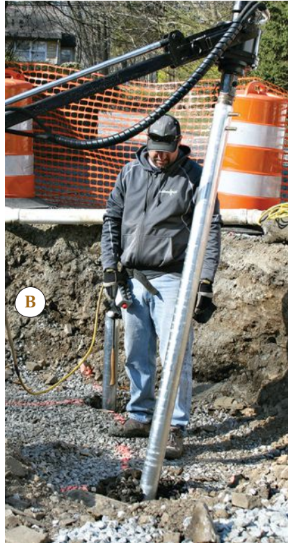
Figure 3. Shaft extensions are welded on and the pier driven as deep as needed to reach soil with adequate bearing capacity (A). The pier can be steered around a below-grade rock by moving the driver's boom; once the obstruction is passed, the boom pulls the shaft plumb again (B). Even though this pier penetrates about 13 feet into the ground, there's no pile of excavated soil as there would be with a conventional footing (C).
