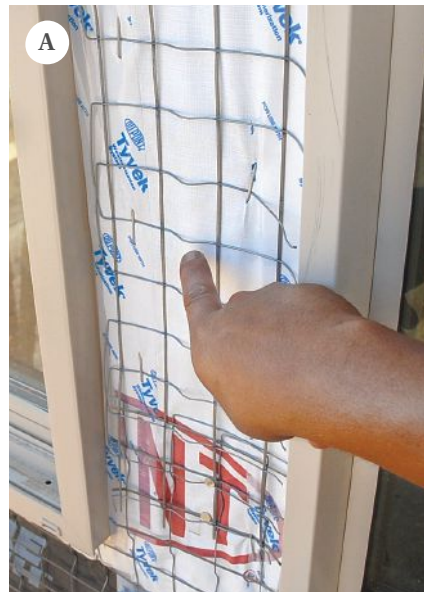
Figure 4. This wire lath (A) has been installed backward; it should be positioned so the ridges hold it away from the wall. The author advises against using staples (B) to attach lath, because the holes they make in the building paper tend to become elongated. Furring nails (C) are preferable; they have a cork washer that holds the wire off the paper and also seals around the shank.
