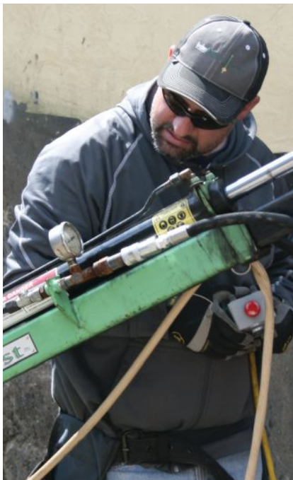
Figure 2. A pier's bearing capacity usually relates to the torque required to drive it. A gauge on the machine measures the hydraulic pressure, which correlates to the torque.
