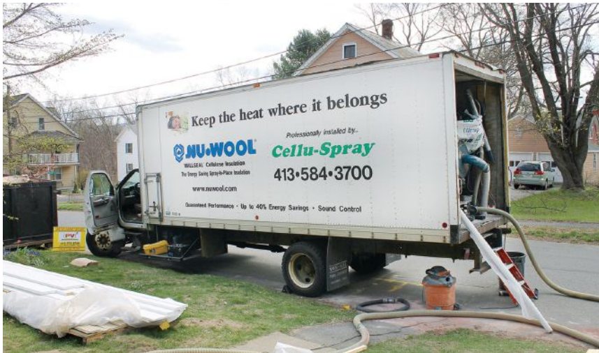
Figure 1. This truck (above) is equipped to install either damp-spray or dense-pack cellulose. The hopper that feeds material to the operator can be filled to the ceiling (right), providing enough material to last from 15 minutes to an hour, depending on the application.
