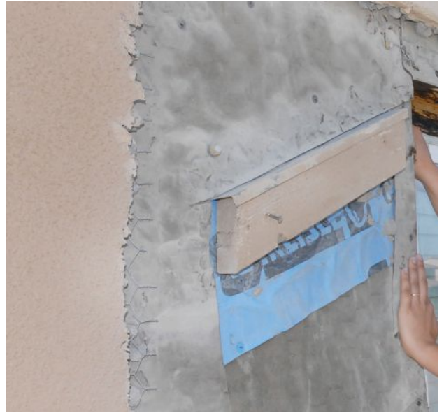
Figure 1. Shown here (above) is a shutter block that was installed on top of a piece of light-blue self-adhered flashing. Unfortunately, the building paper was then installed on top of the flashing beneath the block, which allowed water to run behind the paper and soak the framing. In the repair (right), the flashing membrane sits on top of the paper below the block.
