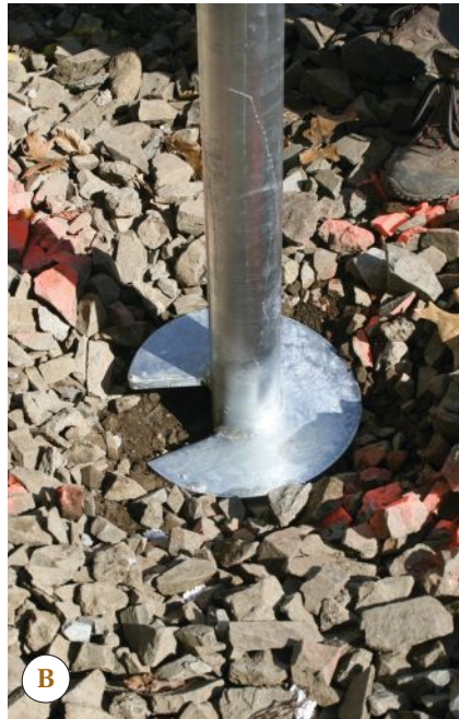
Figure 1. Helical piers have a screw-shaped plate welded to a zinc-coated steel shaft, and are made in different sizes for different soils and applications (A). As the driver turns the pile, it simply screws into the ground until the installer is confident it's below the frostline and in soil with sufficient bearing capacity (B). Several types of caps are available to attach piers to framing; some are adjustable in order to fine-tune the elevation (C).
