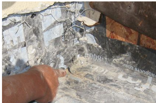
Figure 2. This window's bottom flange was taped to the sheathing (above). Trapped water caused the flashing membrane's adhesive to fail, directing even more water into the framing. Wrinkles in the membranes can also create water paths underneath stucco, as in the wide sill of this recessed window (right).
