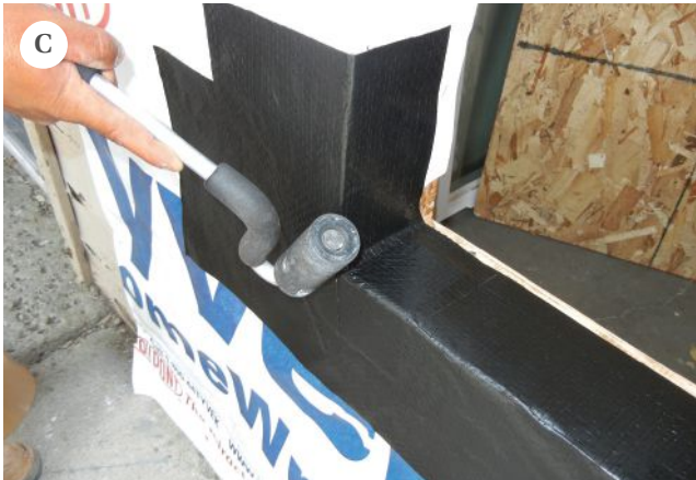
Figure 3. Prefabricated plastic corners (A) and flashing tapes and membranes (B) simplify window and door installation. Always use a roller when installing self-adhering membranes, to get rid of wrinkles (C).
