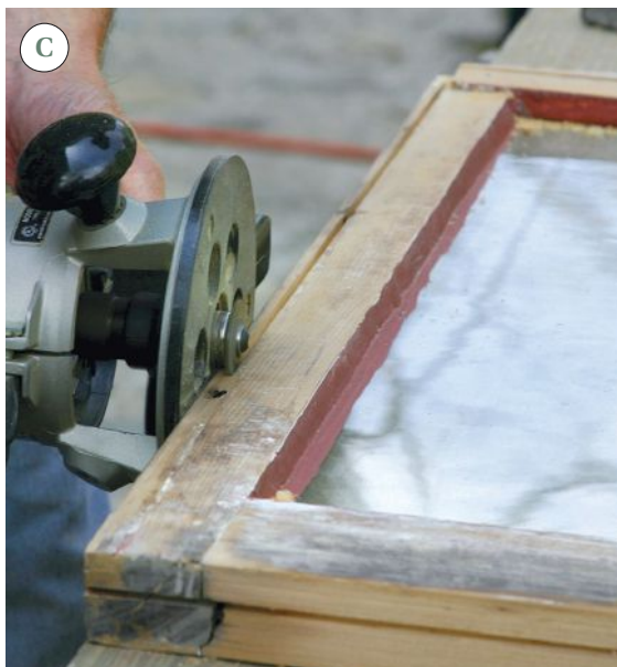
Figure 4. Using a plunge router, the author centers the slot for the bottom tube seal \frac{5}{8} inch from the face of the sash (A); the slot for the meeting-rail seal is centered \frac{3}{8} inch below the top edge (B). The side brush seals are placed as close to the edge as practical — \frac{1}{4} inch (C). Any closer and the thin strip of wood left behind may break off.
