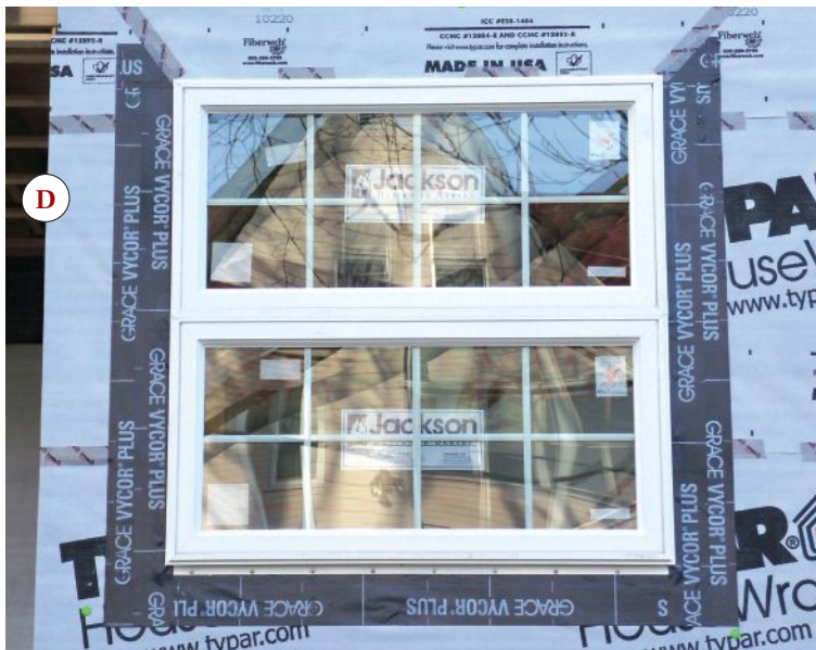
Figure 7. Outer flashing goes on over the window's side and top flanges (A, B). The flap of housewrap above the window head is then pulled down and taped in place over the head flashing (C, D).
