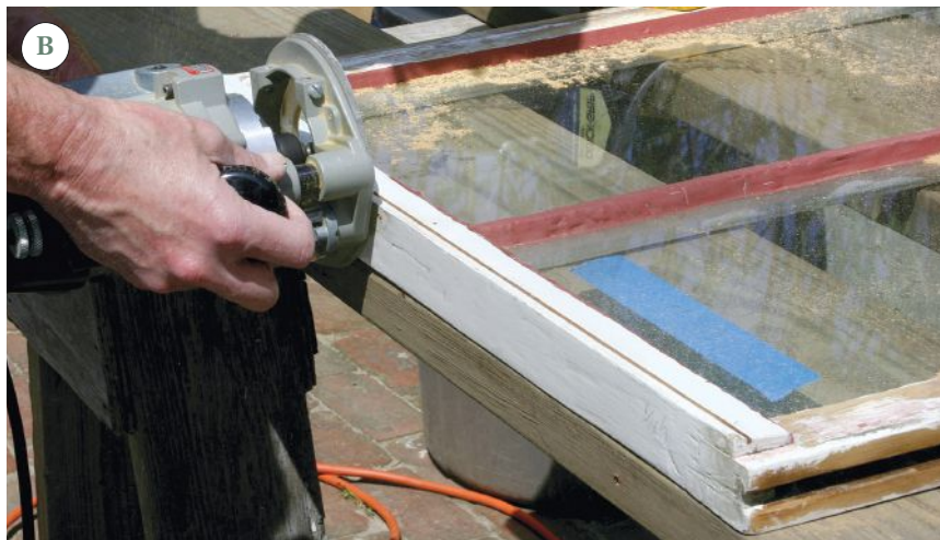
Figure 4. Using a plunge router, the author centers the slot for the bottom tube seal \frac{5}{8} inch from the face of the sash (A); the slot for the meeting-rail seal is centered \frac{3}{8} inch below the top edge (B). The side brush seals are placed as close to the edge as practical — \frac{1}{4} inch (C). Any closer and the thin strip of wood left behind may break off.
