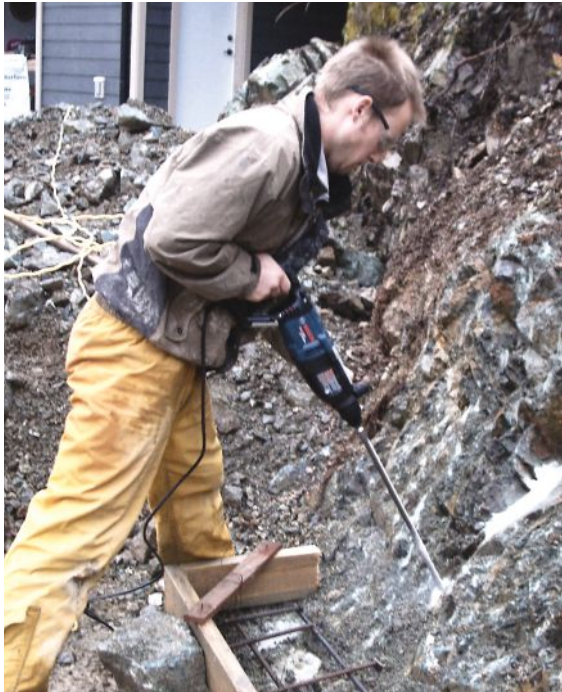
The D-handle tool has a long reach for easier downward drilling.
