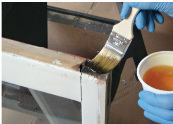
Figure 3. The bottom edge of the sash must be trimmed by about 1/8 inch to account for the thickness of the weather seal (above). After the cut, the end grain gets a treatment of epoxy consolidant to prevent rot infestation (left).
