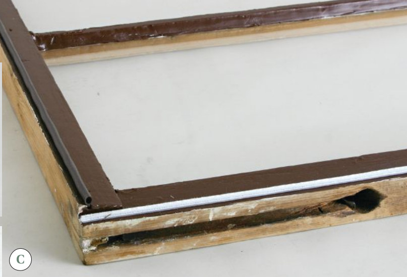
Figure 2. After years of weatherstripping old windows and doors, the author has settled on three seal profiles for most jobs: a polypropylene brush seal for the sides; a 1/4-inch tube seal (white or bronze) for the meeting rail, and a white 3/16-inch tube for the bottom (A). Slots for the seals are cut with a 3-millimeter slot cutter (B); the seals are installed with a screen tool or by hand (C).
