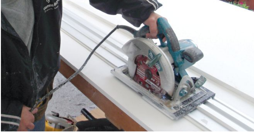
Figure 8. The author uses a track saw to create exterior trim of any width from 3/4-inch PVC sheet stock.
