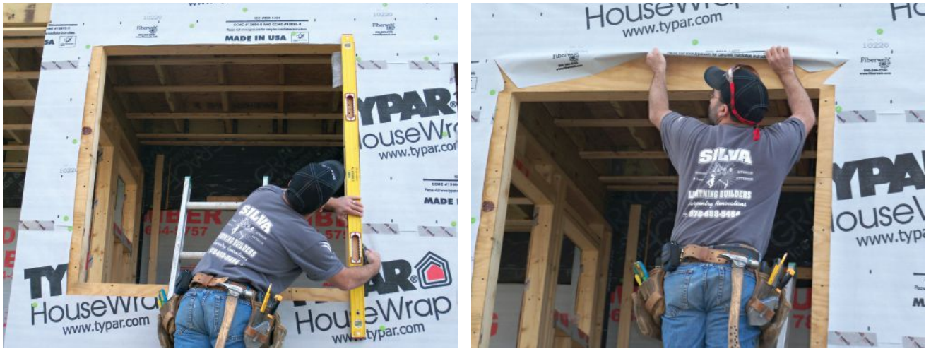
Figure 1. Once the housewrap has been cut back from the sides and bottom of the rough opening by the width of a level (left), a flap along its upper edge is temporarily tucked out of the way (right).
