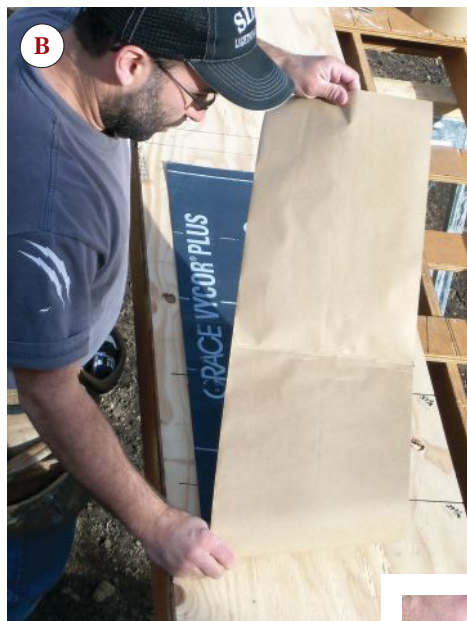
Figure 2. Transferring the dimensions of the flashing pieces to a plywood story board makes it easier to cut them accurately to length (A). Each piece is then folded lengthwise twice (B) so it's short enough to cut against a standard framing square (C). Corner pieces, or bow ties — measuring about 1½ inches by 8 inches overall — are cut from scrap material (D, E).
