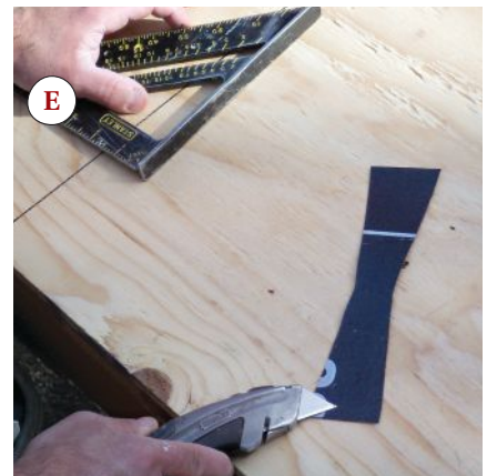
Figure 2. Transferring the dimensions of the flashing pieces to a plywood story board makes it easier to cut them accurately to length (A). Each piece is then folded lengthwise twice (B) so it's short enough to cut against a standard framing square (C). Corner pieces, or bow ties — measuring about 1½ inches by 8 inches overall — are cut from scrap material (D, E).
