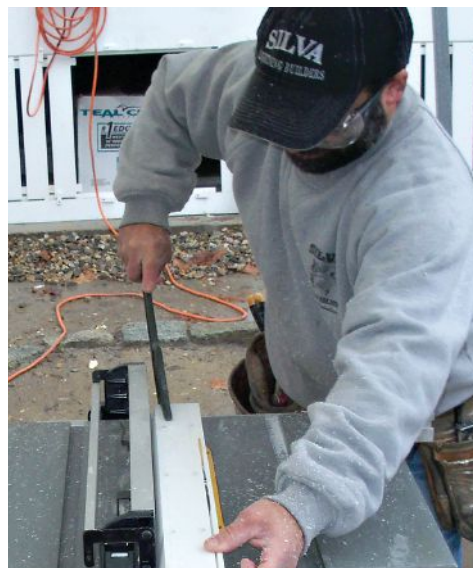
Figure 8. The author uses a track saw to create exterior trim of any width from 3/4-inch PVC sheet stock.
