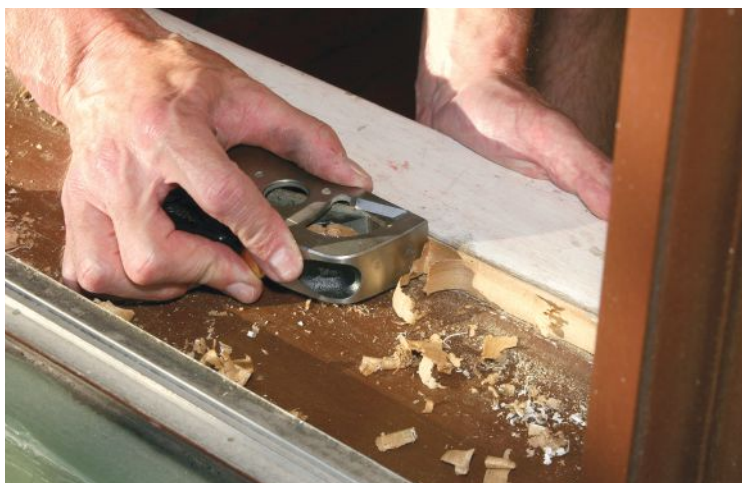
Figure 5. Before the weatherstripped sash can be reinstalled, the stool must be scribed and trimmed to allow for the thickness of the brush seals on the face of the side rails. A \frac{1}{16} -inch-wide gap, scribed with a carpenter's pencil, allows for expansion (top). A bullnose plane with a removable toepiece cuts away the excess stock with a minimum of dust (above).
