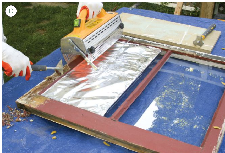
Figure 1. A lead-safe work zone is needed when working with old double-hungs (A). A spring clamp prevents the sash cord from dropping into the pocket; on the window shown (B), the trim was in bad shape and was removed for replacement, allowing the author to insulate the cavity with XPS and spray foam. To improve the window's operation, old paint is removed from all running surfaces; here the author uses an infrared paint-stripping tool (C). Paint is also removed from the inside of the window frame and the edge of the stop (D); raw wood surfaces will be waxed.
