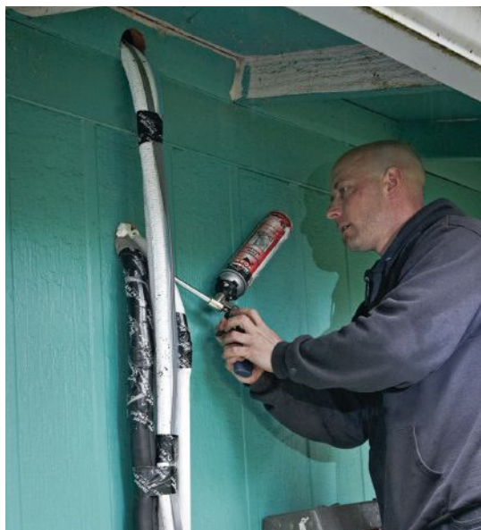
Figure 5. After the mounting bracket of a wall-mounted indoor unit is screwed to the studs (top), the unit itself is hung on the bracket, with the stubs for refrigerant lines, a condensate drain, and an electric line passing through a hole in the exterior wall (center). The 2 9 / 16 -inch hole is later filled with canned closed-cell foam and waterproofed with caulk (above).
