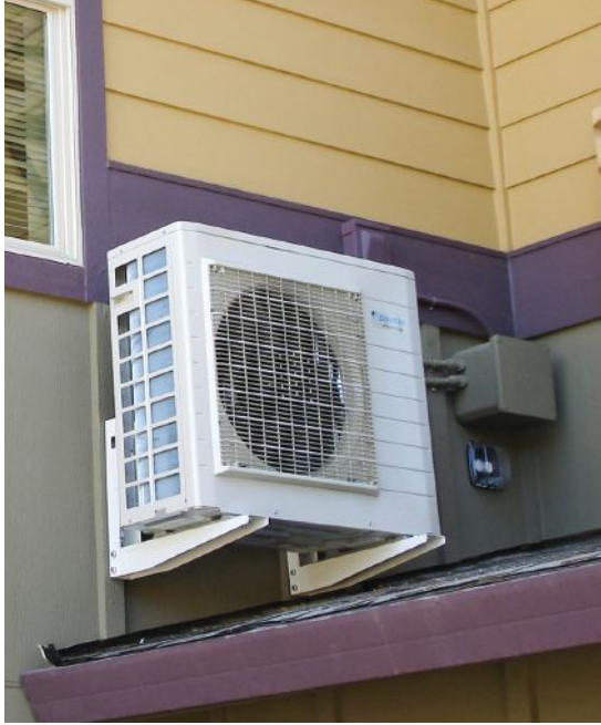
Figure 7. If no suitable position for a ground mount is available, the unit can be wall-mounted on a manufactured bracket.
