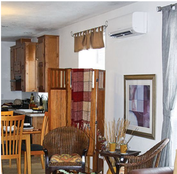
Figure 1. Ductless heat pumps deliver cooled or heated air with one or more indoor fan-coil units. For this home's single-zone system, the surface-mounted indoor unit has been placed in a central area of the living space to distribute the conditioned air as widely as possible.
