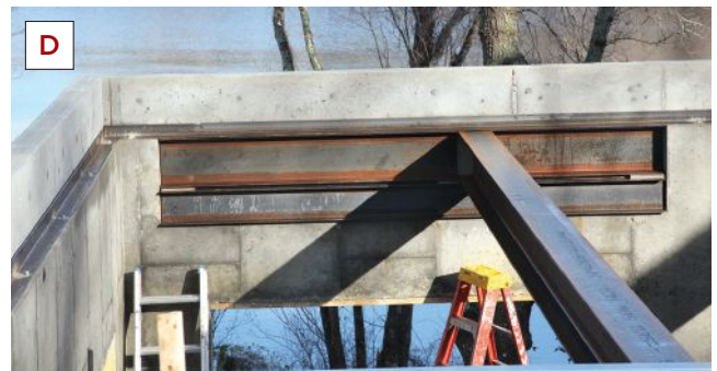
Figure 2. I-beams provide midspan support for the garage floor. A header beam spans the door opening at the rear of the building (A) and also supports one of the I-beams (B). The second beam sits in the formed foundation pockets (C). Sections of steel channel shimmed to the correct elevation on top of the header support the perimeter steel angle (D).
