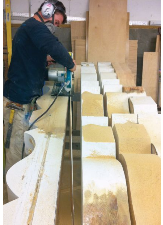
Figure 2. The new and old column sections were joined together with galvanized through-bolts and epoxy (above). Once the columns were reassembled, a worker straightened them with a large-capacity beam saw (right).
