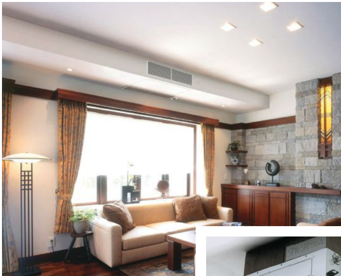
Figure 4. Although indoor units are most often mounted high on a wall, some models are designed to be concealed in a soffit (above) or mounted flush in a dropped ceiling (right). Floor-mounted low-wall units (far right) are also available.
