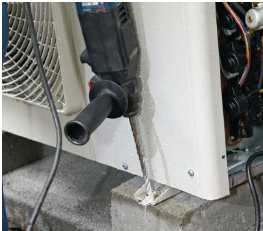
Figure 6. Concrete riser blocks — which elevate the outdoor unit to provide drainage — are fastened to the pad with construction adhesive (top). Then the outdoor unit itself is put in position (center) and fastened to the risers with Tapcon screws (above).
