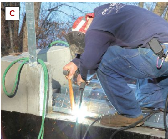
Figure 3. A worker bolts the steel angle to the perimeter shelf (A), then the crew sets the steel pans, which are strong enough to walk on but light enough to carry easily (B). A welder then spot-welds the pans to the perimeter angle (C) and the I-beams (D).
