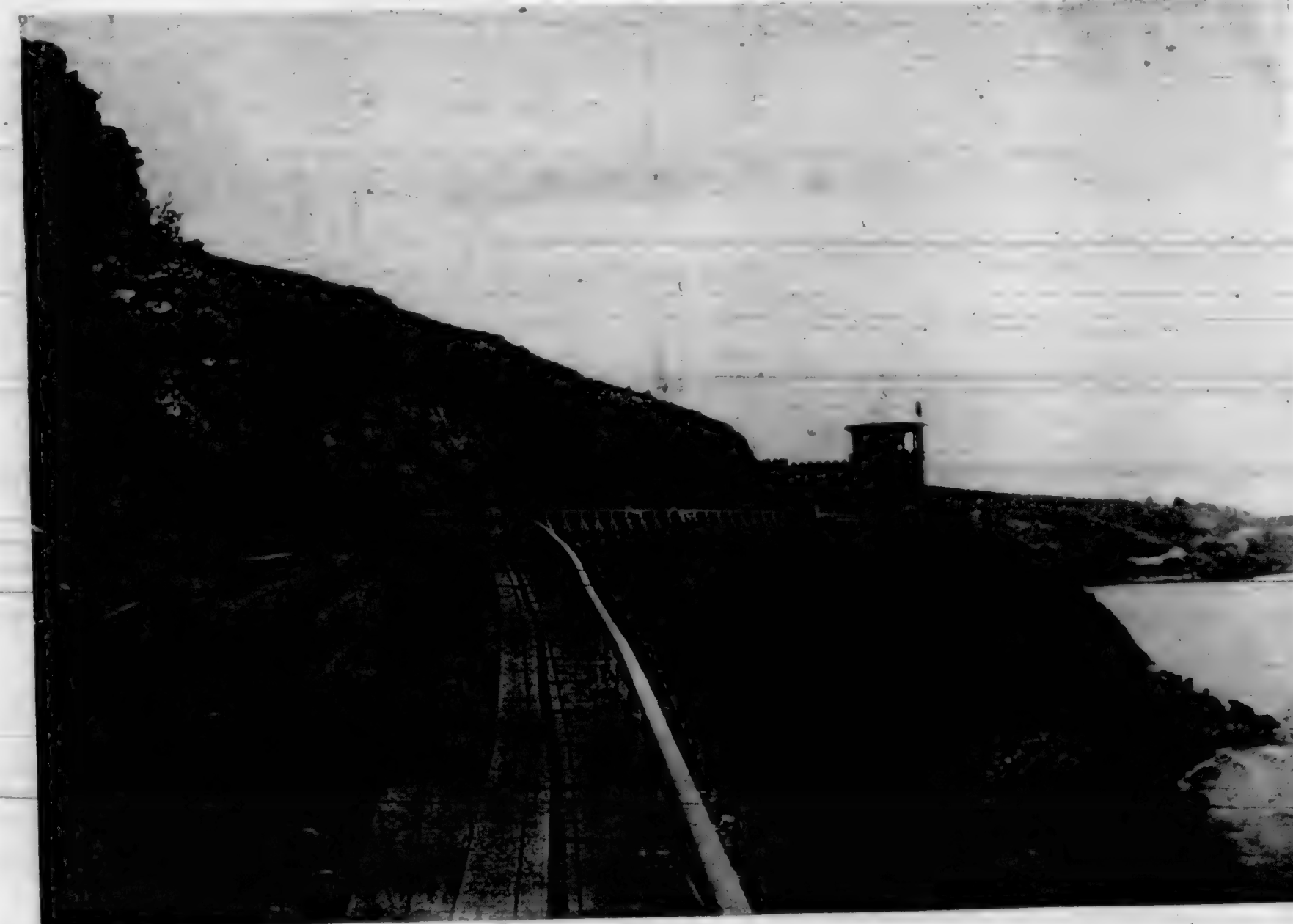
ROADWAY ALONG THE ROCKY SHORE AT TIBURON
