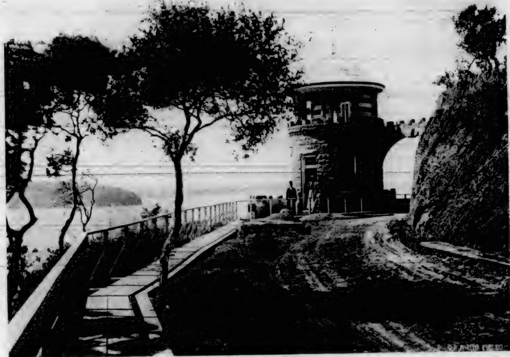
THE GATEWAY AND WATCH TOWER AT POINT TIBURON.
