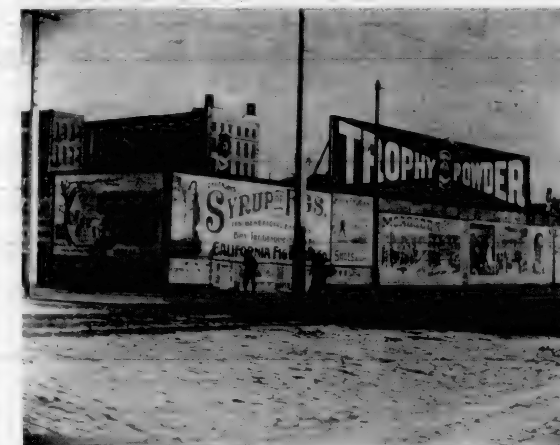
PREMISES OF NEW SAN FRANCISCO POST-OFFICE, AUTHORIZED BY ACT OF CONGRESS, MARCH, 1887.
