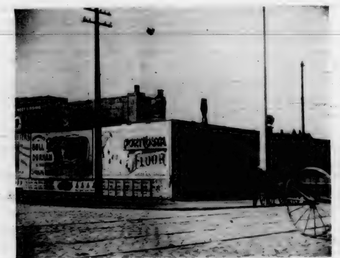
PREMISES OF NEW SAN FRANCISCO POST-OFFICE, AUTHORIZED BY ACT OF CONGRESS, MARCH, 1887.
