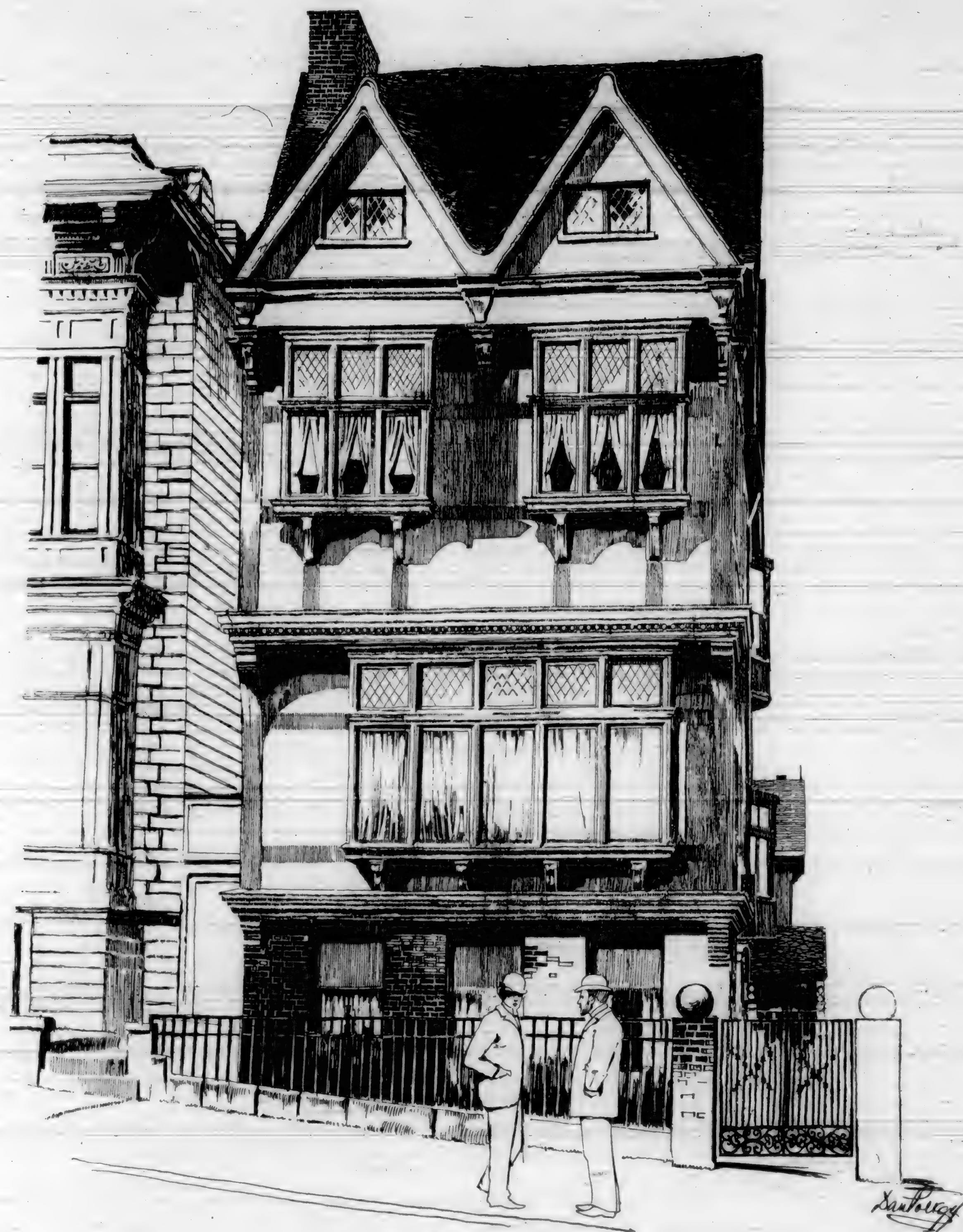
DR. BOERICKES' HOUSE ON WASHINGTON STREET SAN FRANCISCO. POLK AND GAMBLE ARCHITECTS.
