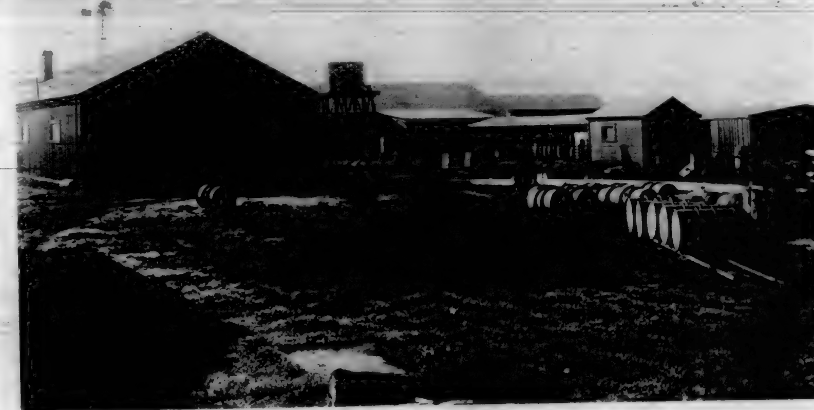
PAINT FACTORY AND STORAGE SHEDS OF PARAFFINE PAINT CO., AT BERKELEY, CAL.
