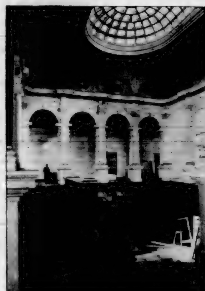
INTERIOR OF DOME, MUSEUM.
