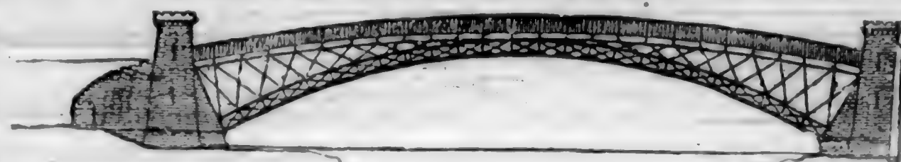
CAST IRON BRIDGE AT CRAIGELLACHIE.
