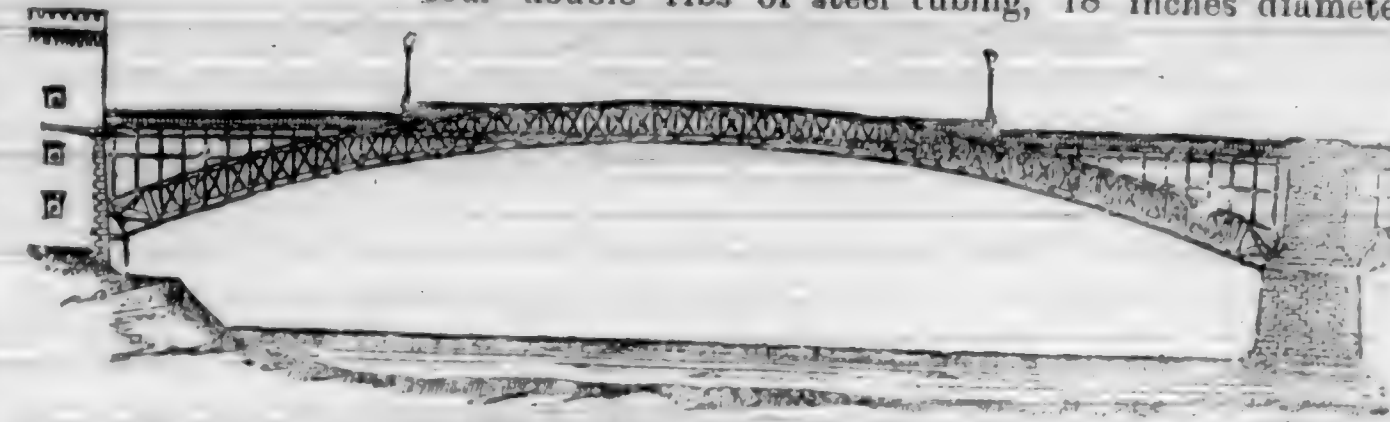
ARCH BRIDGE AT COBLENTZ.
