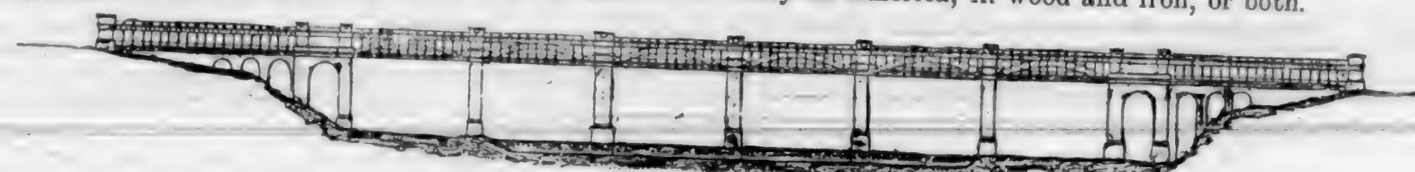
HIGH LEVEL BRIDGE AT NEWCASTLE.
