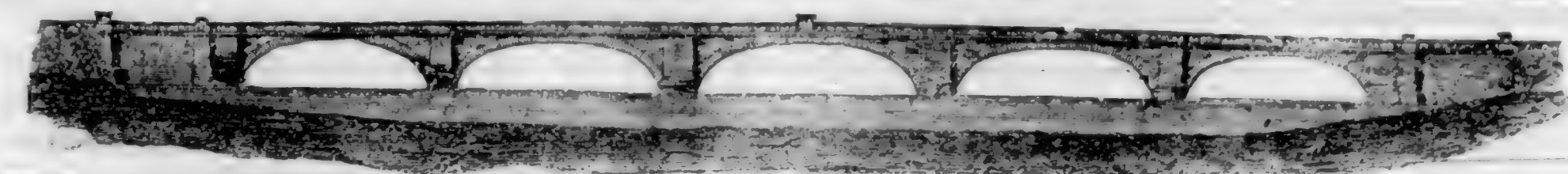
LONDON NEW BRIDGE.
