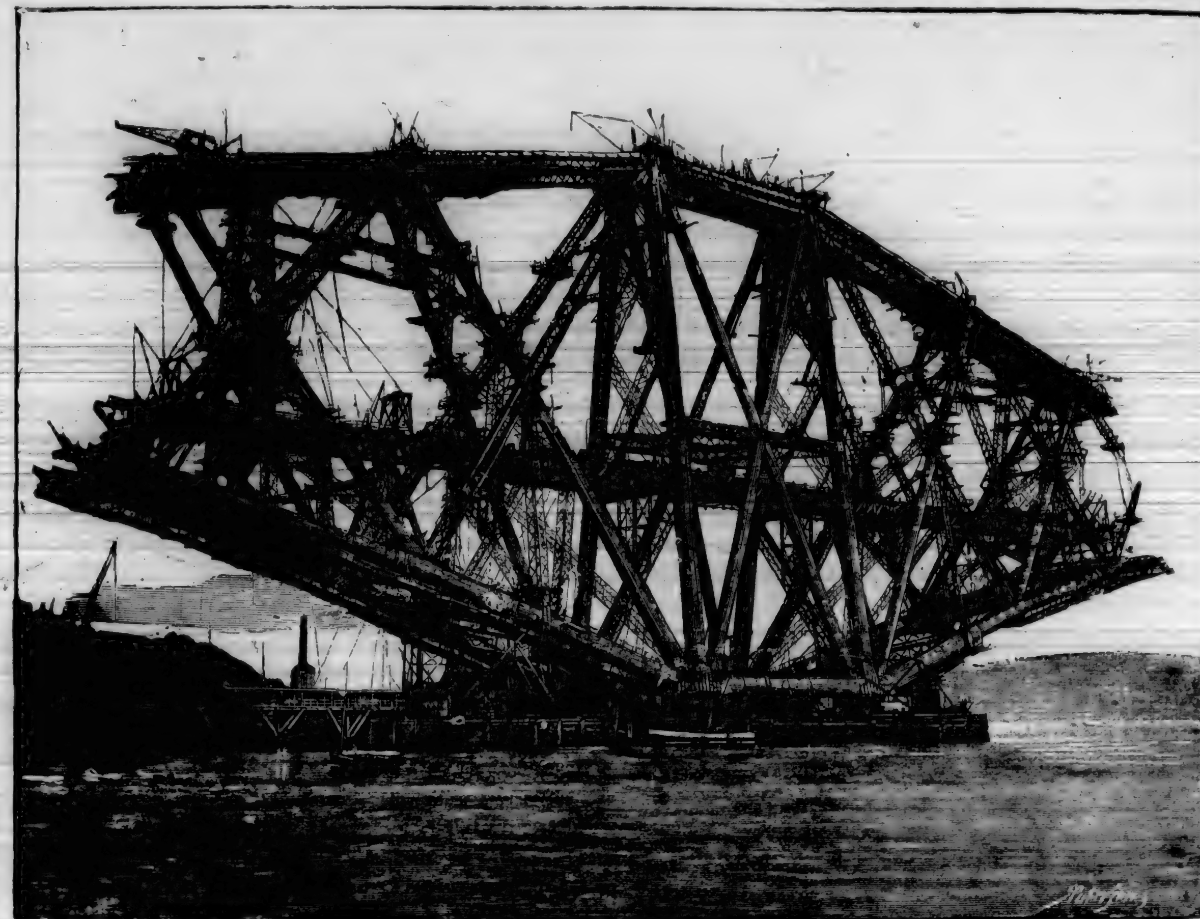
FIRTH OF FORTH CANTILEVER BRIDGE.
