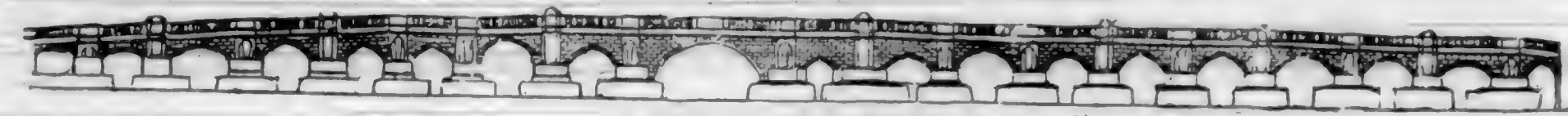
LONDON OLD BRIDGE.
