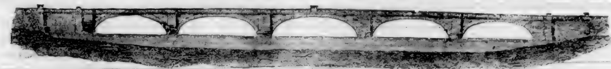
LONDON NEW BRIDGE.
