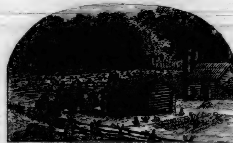
THE LOG HOUSE.
